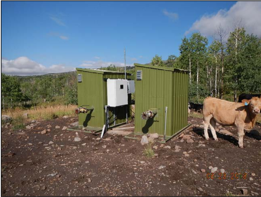
Photo 3. Disconnected separators.
