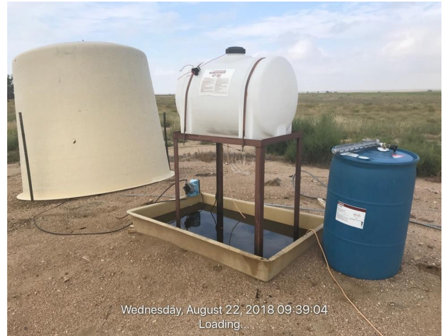
Photo#2 Corrective action/Containment needs cleared out and blue barrel needs to be put into containment
