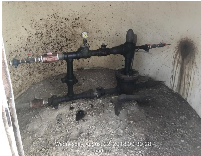
Photo#3 Wellhead/Corrective Action Stained soil and sprayed oil needs cleaned up
