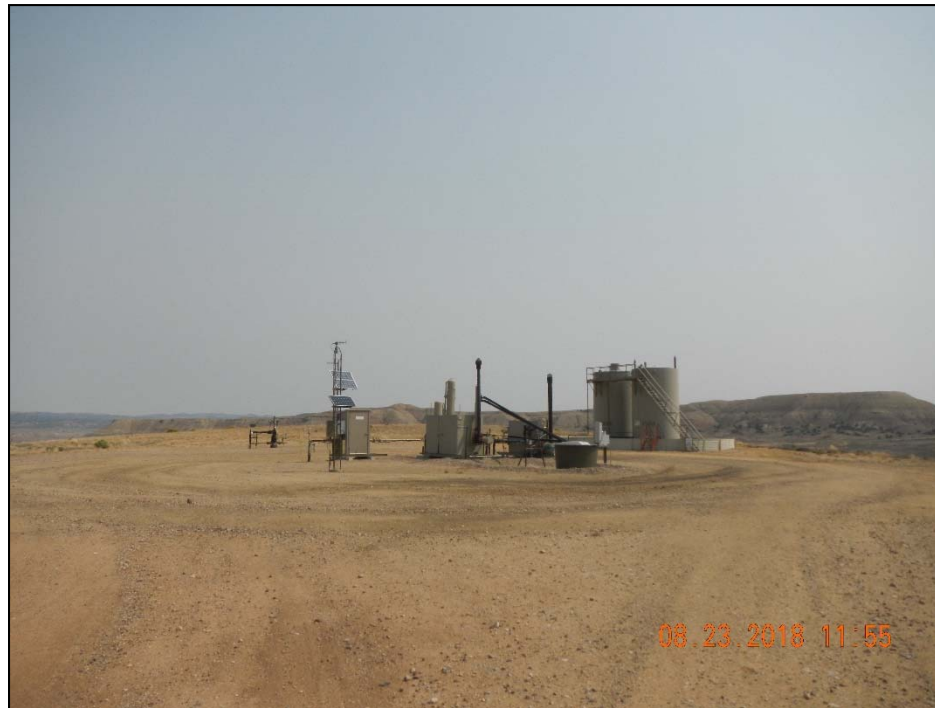
Photo 1. Overview of location taken at entrance facing northeast.
