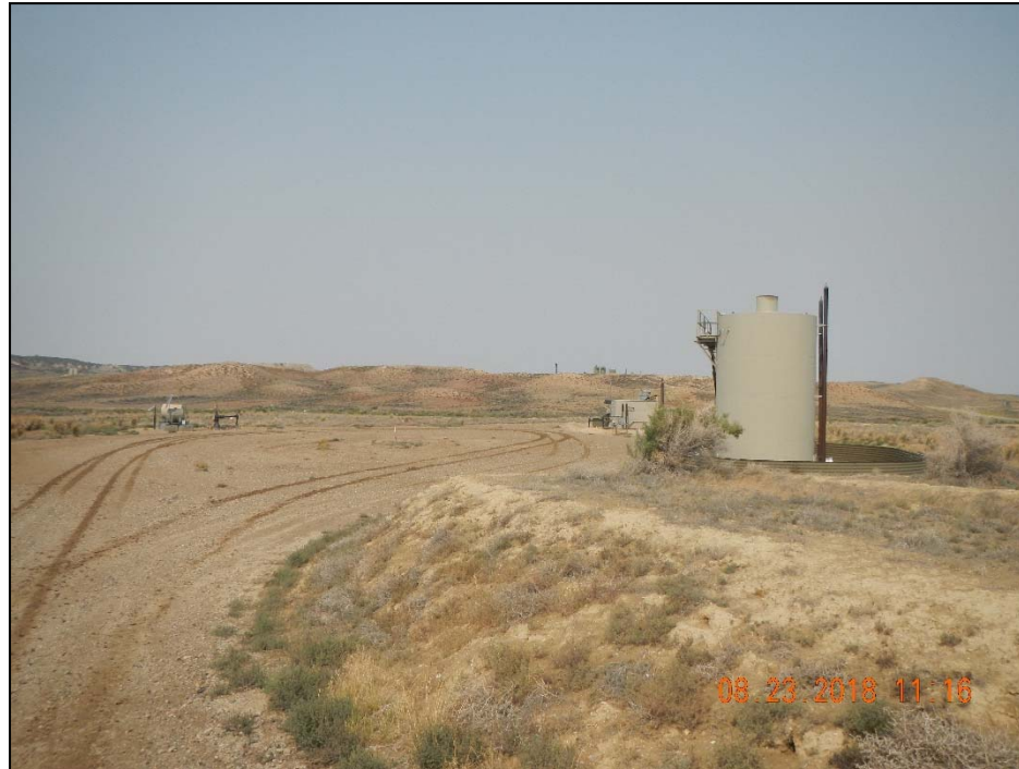
Photo 1. Overview of location taken at entrance facing southwest.
