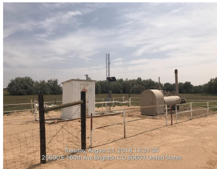
Photo#2 Separator and Gas Meter
