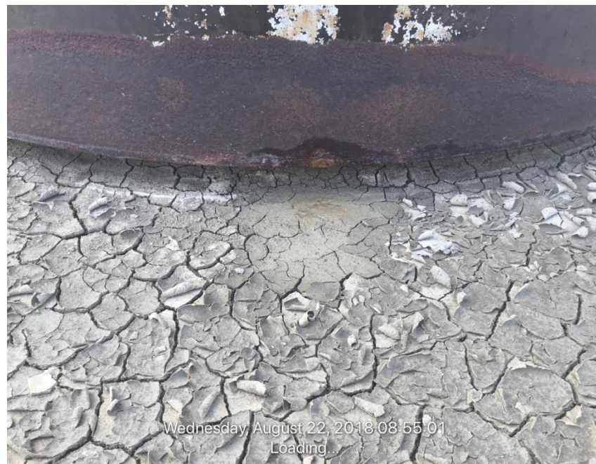
Photo#2 Corrective action Hole in bottom of production tank
