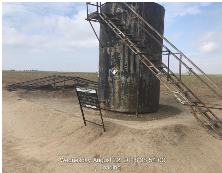
Photo#1 Production Tank/Corrective action Berm in disrepair/Labeling for what is in tank needs to be fixed
