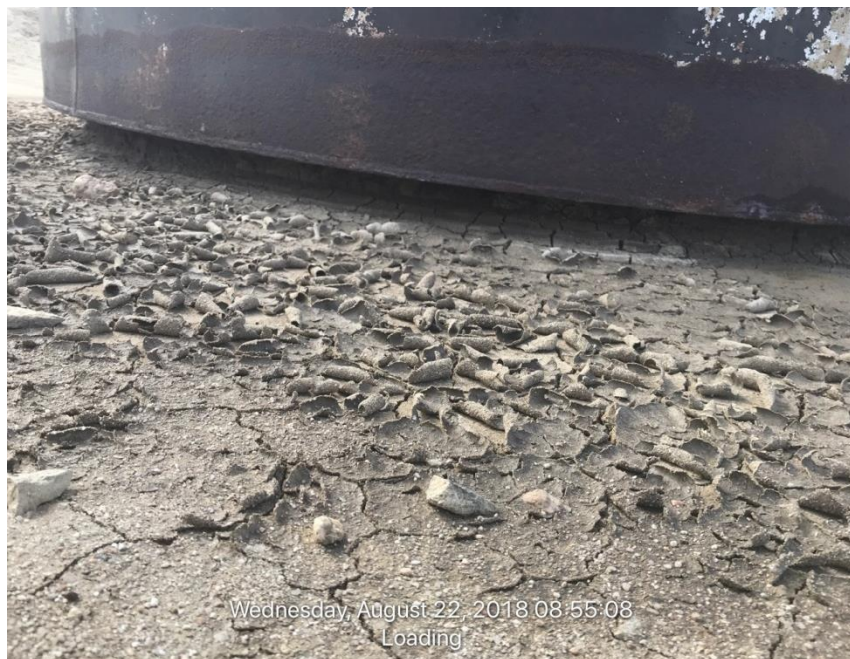
Photo#3 Corrective Action underneath of tank needs to be filled in.
