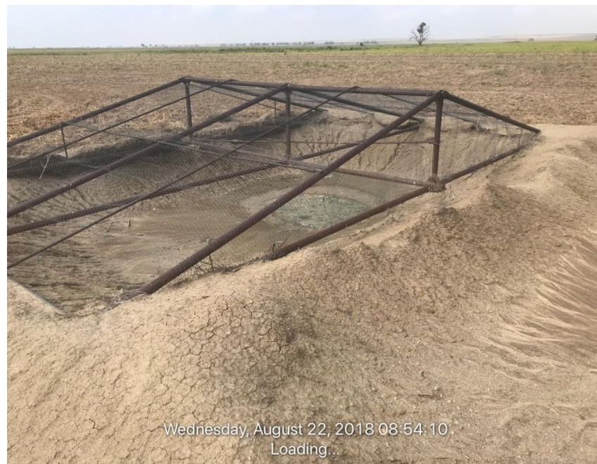
Photo#4 Pit/Corrective Action many openings around frame and screen. Needs to be fixed to prevent wildlife from entering
