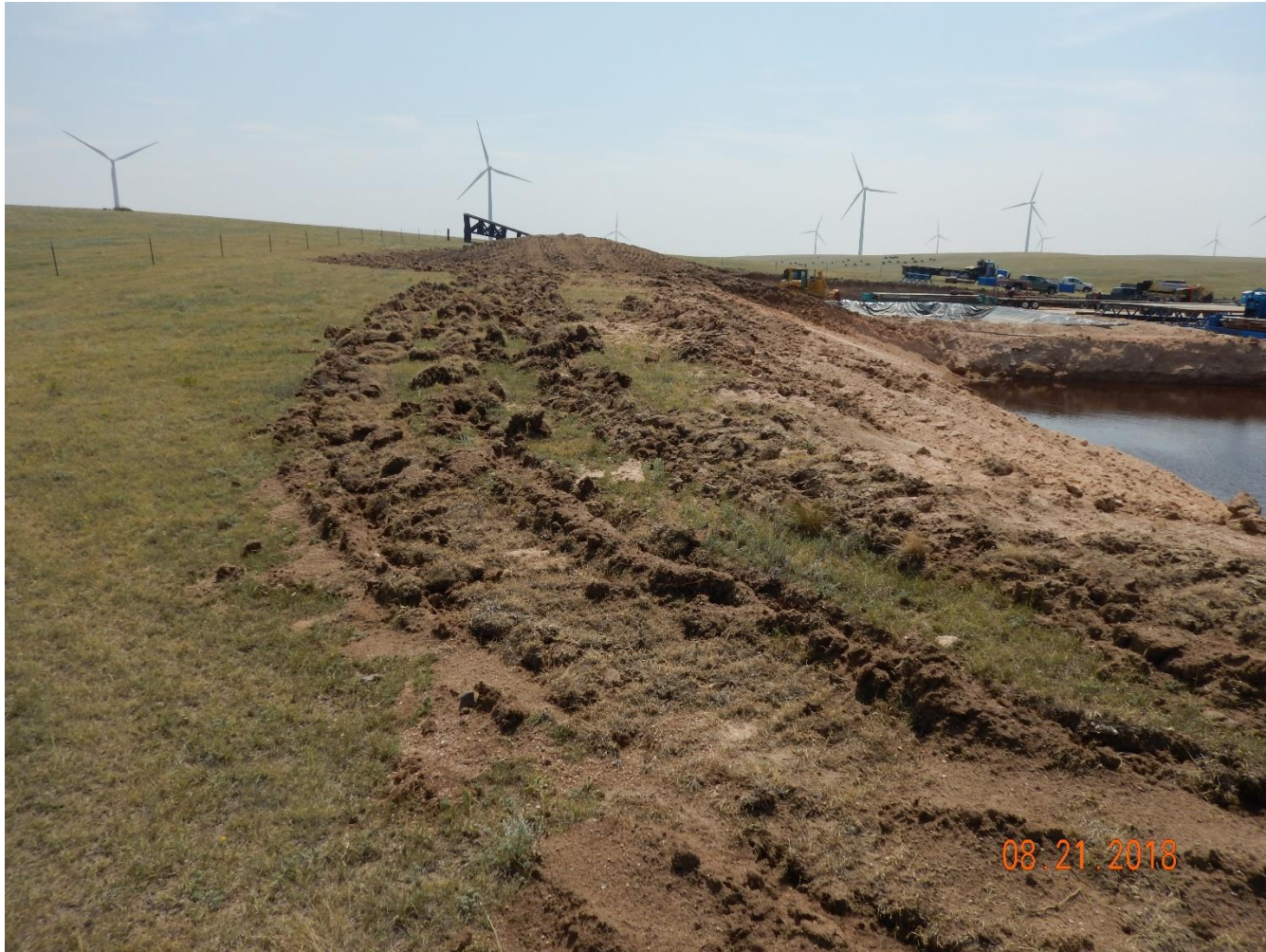
Photo 20: Photo taken from the southeast corner of the location, facing north. Photo shows surface roughening (ripping) has been used in conjunction with a ditch and berm on the east end of the location. . It is noted that the ditch and berm appear to have been constructed with topsoil from the location. This should be avoided to mitigate potential compaction concerns in the topsoil.
