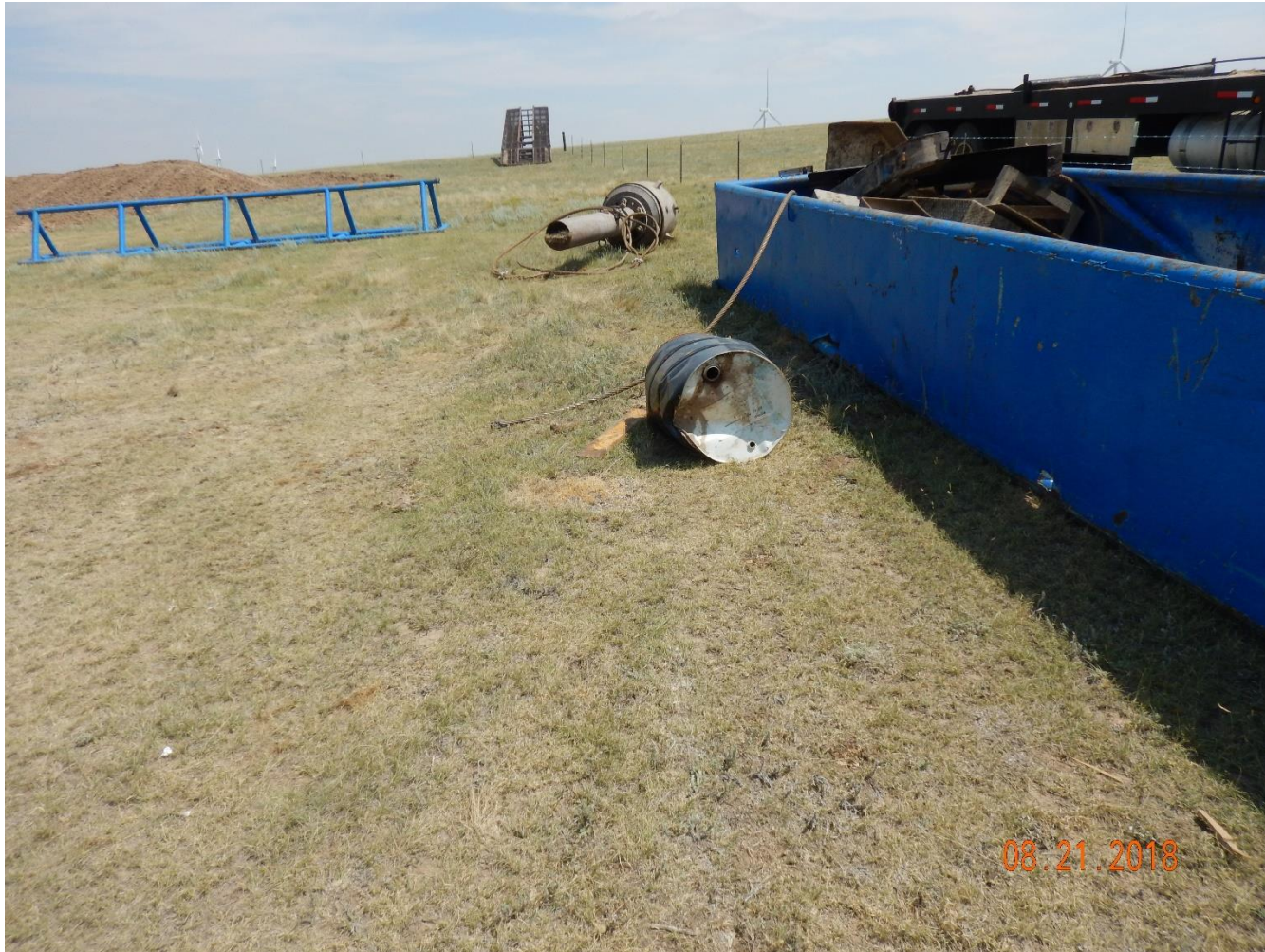
Photo 28: Photo taken from the south end of the location, facing north. Photo shows equipment being stored off the constructed pad. Photo also shows an open barrel laying on its side upon the soil surface. This is improper storage of material and material management. Barrel needs to be placed in secondary containment or removed and properly stored or disposed. Any contaminated soils will need to be cleaned/remediated or removed and properly disposed.
