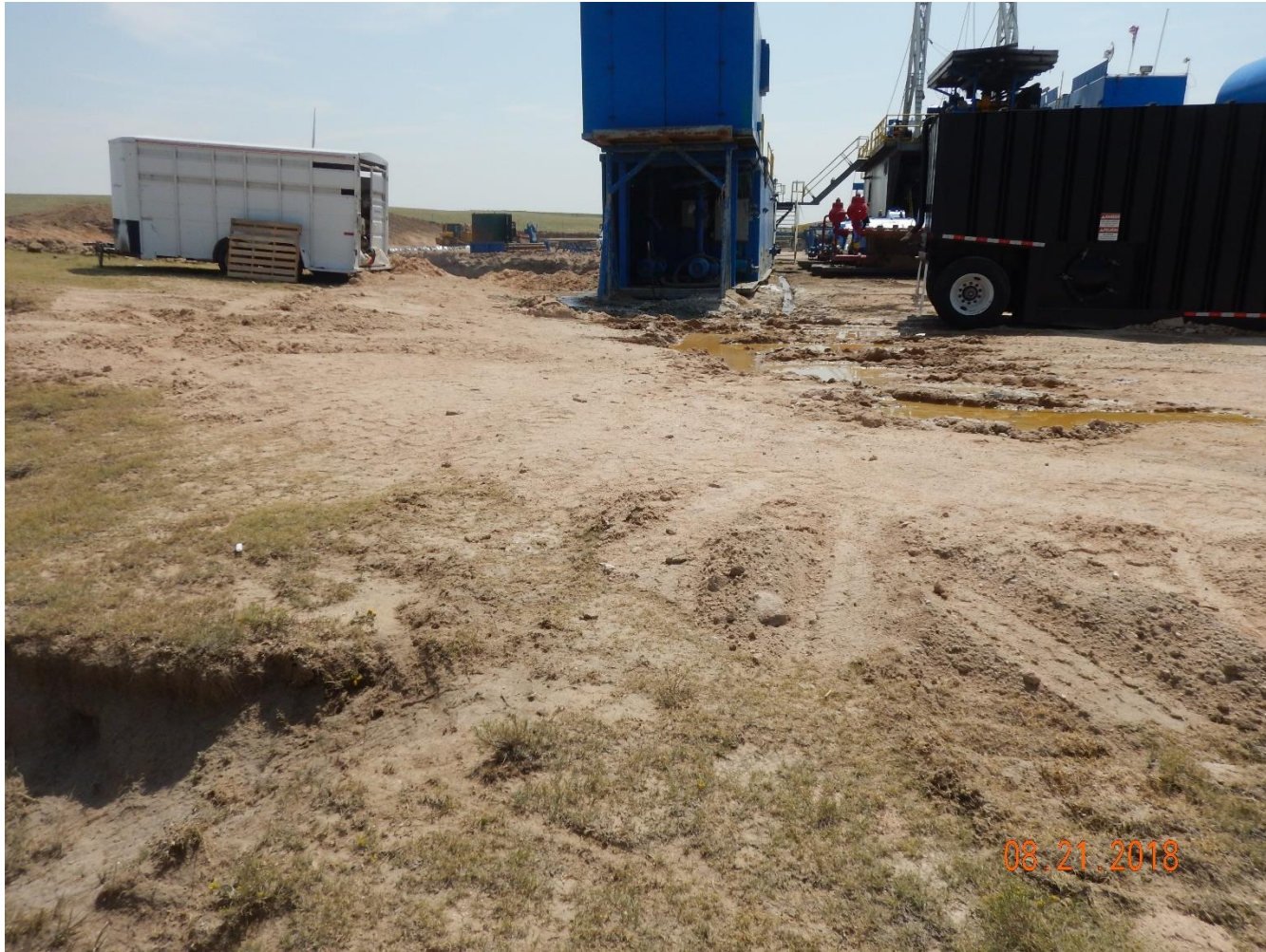
Photo 12: Photo taken from the north end of the location, facing south photo shows various fluids/chemicals from drilling operations ponding on then north end of the pad. Photo also shows the beginning of a drainage to the north of the location (see photo 43). COA in 2A doc. #401333215 states "Location lies within proximity to a tributary of the Lickdab Creek and 275 feet from Lickdab Creek. Operator shall use engineering controls and best management practices to mitigate potential contaminant, including sediment, migration into the nearby surface waters". Photo shows no stormwater or erosion controls have been installed on the north end of the location.
