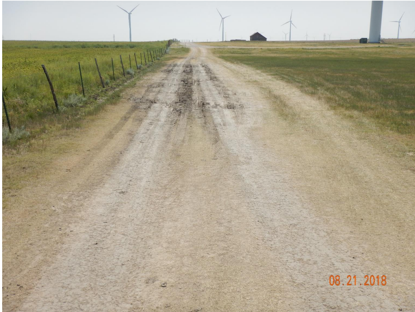
Photo 42: Photo taken from the access road, south of the location, facing south. Photo shows areas of the access road where rutting as occurred. Photo also shows evidence of vehicular travel off of the access road. Maintenance should be conducted and BMPs implemented to allow for travel along access road and minimize off-location/road disturbances in accordance to 1002.e(4)
