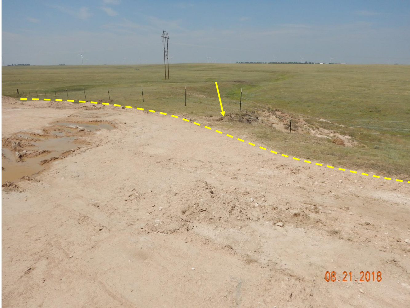
Photo 18: Photo taken from the north end of the location, facing southwest. Photo shows equipment and fluids/chemicals on the pad. See comments under photo 15. Photo also shows area where the pad ends and the beginning of the drainage to the north. Photo shows to stormwater or erosion control BMPs have been installed on the north end of the location.
