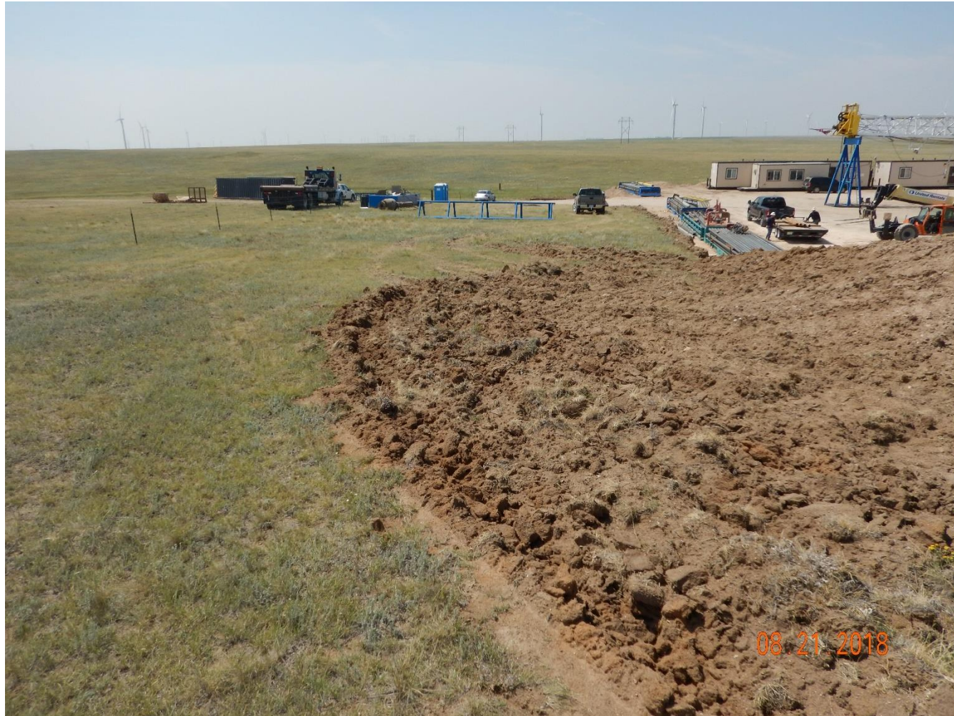
Photo 24: Photo taken from the southeast corner of the pad, facing west. Photo shows stormwater and erosion controls have only been partially installed on the south end of the location.
