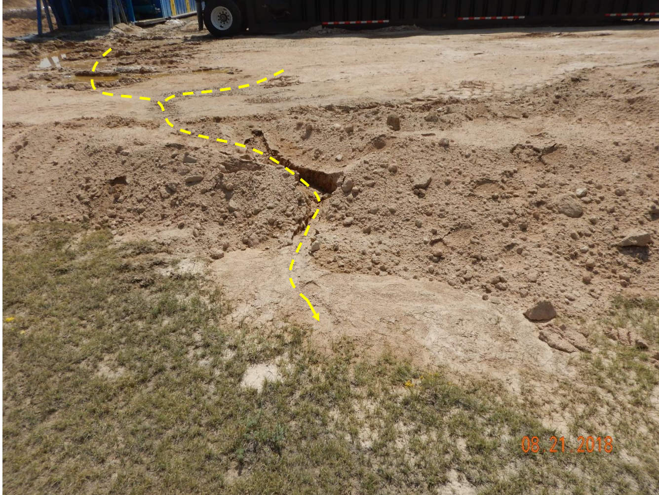
Photo 19: Photo taken from the north end of the location. Photo shows erosion degradation and sediment transport off location from stormwater discharge. Photo also shows water movement patterns from the location.
