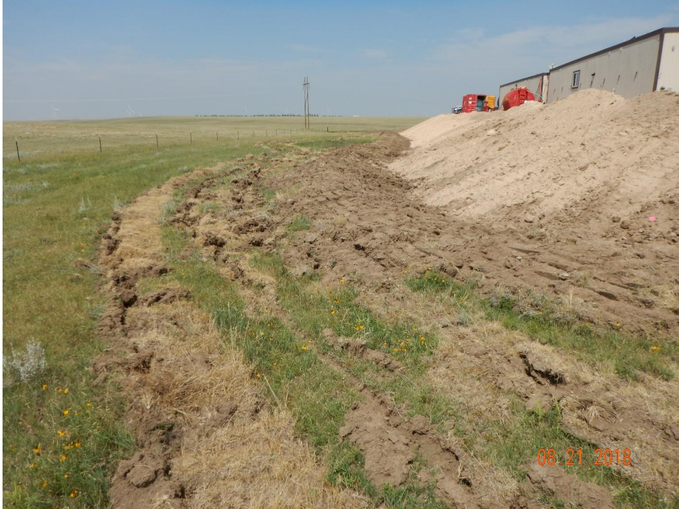
Photo 7: Photo taken from the southwest corner of the location, facing north. Photo shows surface roughening (ripping) has been used in conjunction with a ditch and berm. It is noted that the ditch and berm appear to have been constructed with topsoil from the location. This should be avoided to mitigate potential compaction concerns and sediment loss in the topsoil.
