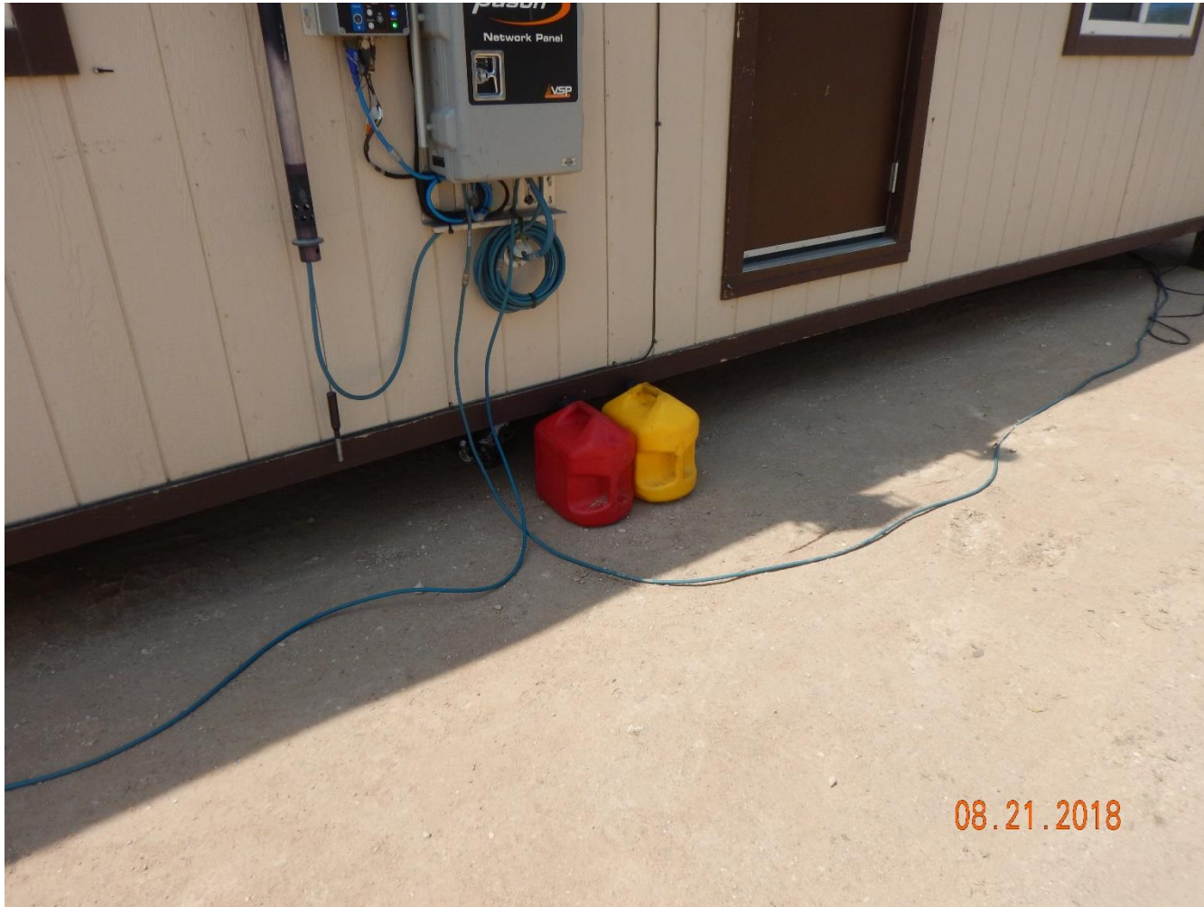
Photo 33: Photo taken from the west end of the location adjacent to the trailers on site. Photo shows gas cans improperly stored on location. See comments under photo 28.
