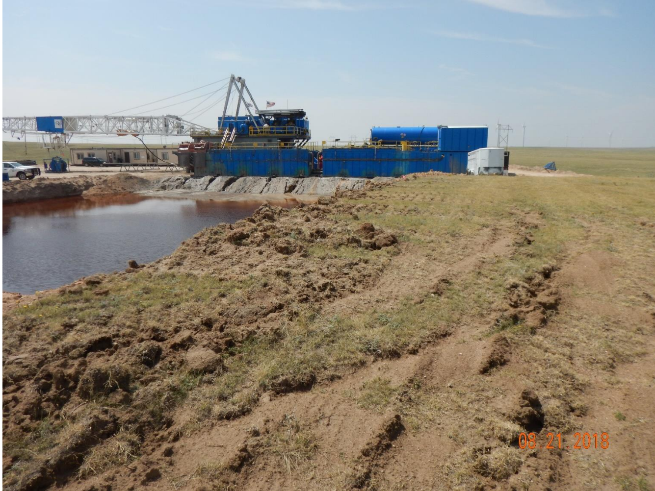
Photo 21: Photo taken from the northeast corner of the location, facing west. Photo shows drill rig, production pit. Photo also shows nor stormwater and erosion control BMPs have been installed on the north end of the location.
