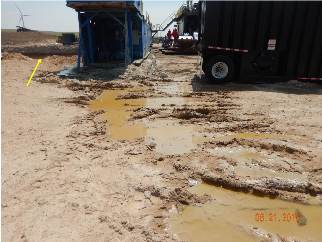
Photo 15: Photo taken from the north end of the location, facing south. Photo shows various fluids/chemicals from drilling operations ponding on then north end of the pad. Fluids appear to be traveling north from the drill rig, equipment and the intended production pit (arrow)
