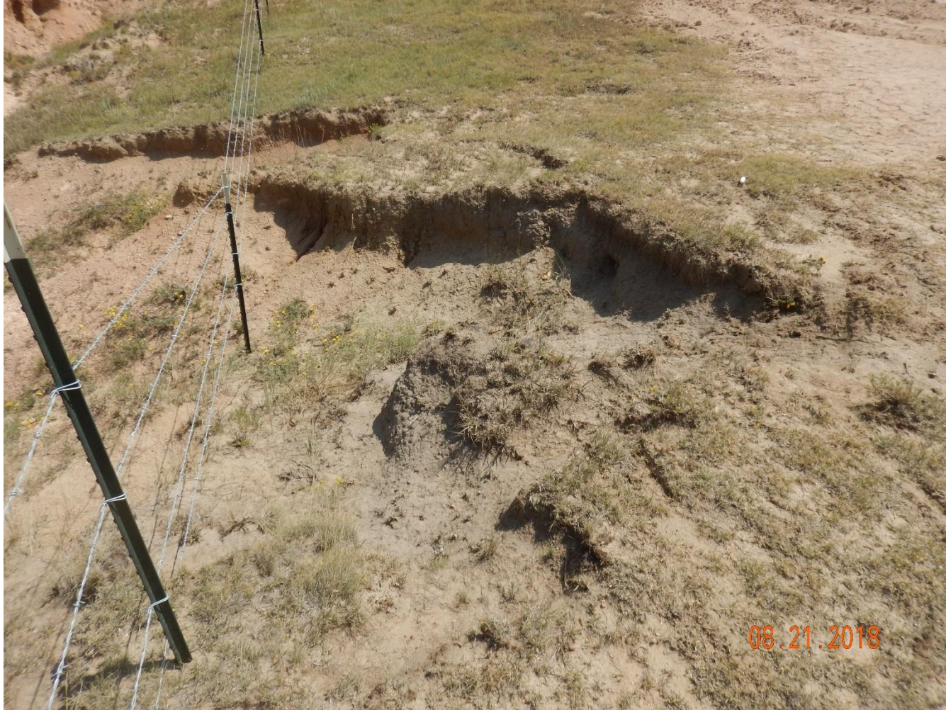
Photo 13: Continued from photo 12. Photo shows drainage. It is noted that the drainage is approximately 3-5 feet from the pad. Photo shows not stormwater or erosion controls have been installed on the north end of the location.
