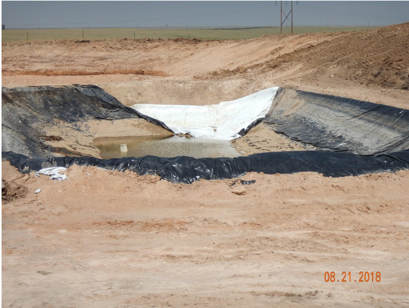
Photo 27: Photo taken from the south end of the location, facing north. Photo shows liner within pit is not in proper functioning condition.
