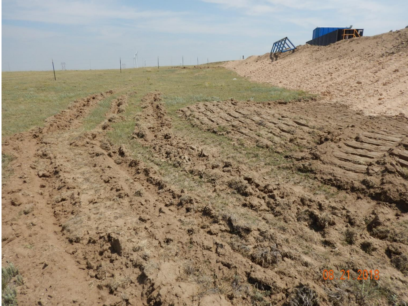
Photo 10: Photo taken from the northwest corner of the location, facing east. Photo shows perimeter controls do not continue on the northern perimeter of the location.
