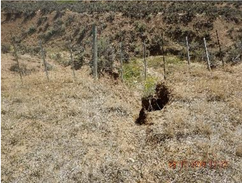
Photo 5: Erosion gulley off SE slope.
