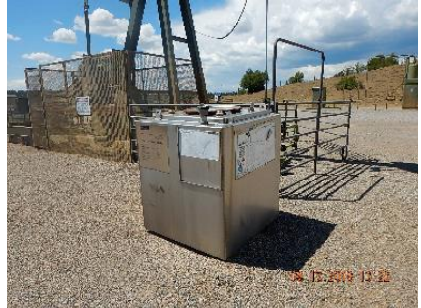
Photo 2: Faded unreadable labels on chemical tank containment.
