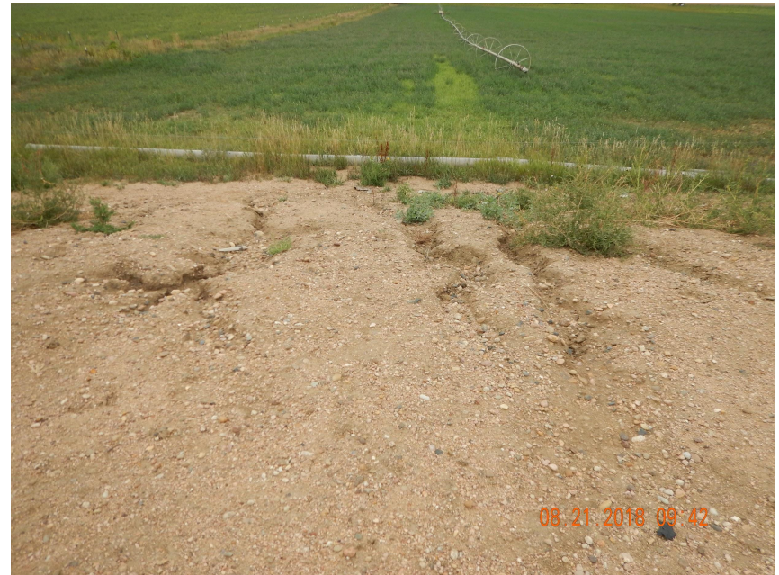
Photo 2. Photo taken from the western fill slope of the tank battery location, facing West. Photo illustrates rill erosion along the fill slope.
