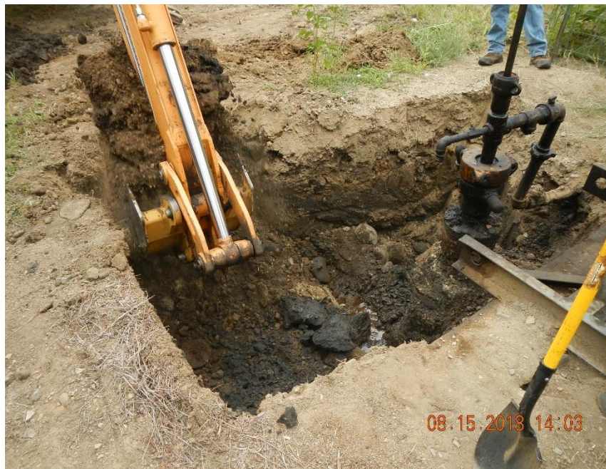
Material being removed from north side of well head.
