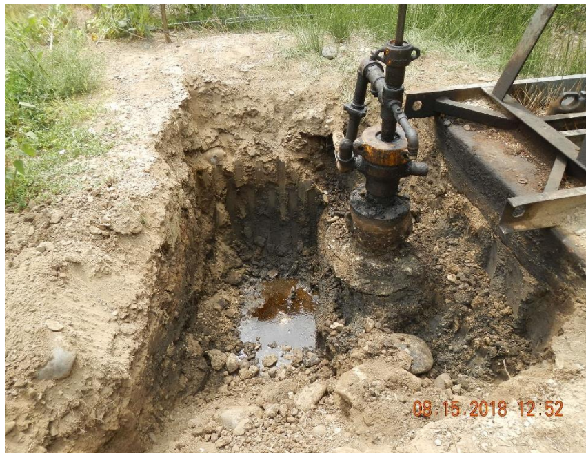
Excavation became wet at approximately 4' bgs.
