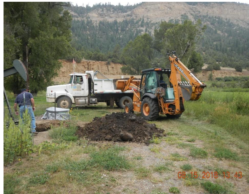
Stained soil being loaded onto 12 cy dump truck.
