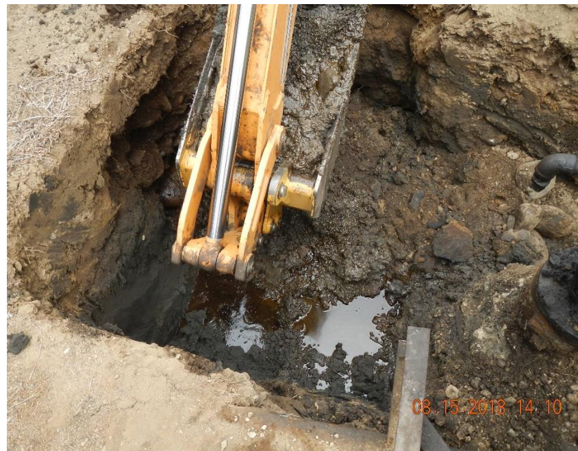
Excavation of stained soil with infiltration of ground water.
