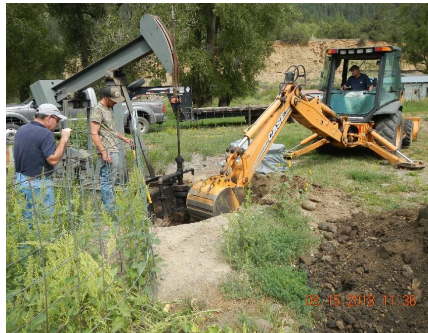
Rivas Earthworks beginning to excavate impacted soil from around the Chavez #1 well head.
