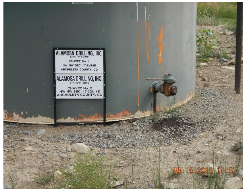
Impacted soil remains underneath truck load out valve on AST.
