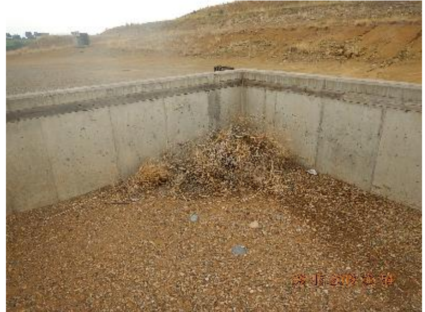
Photo 4: Debris inside tank containment.
