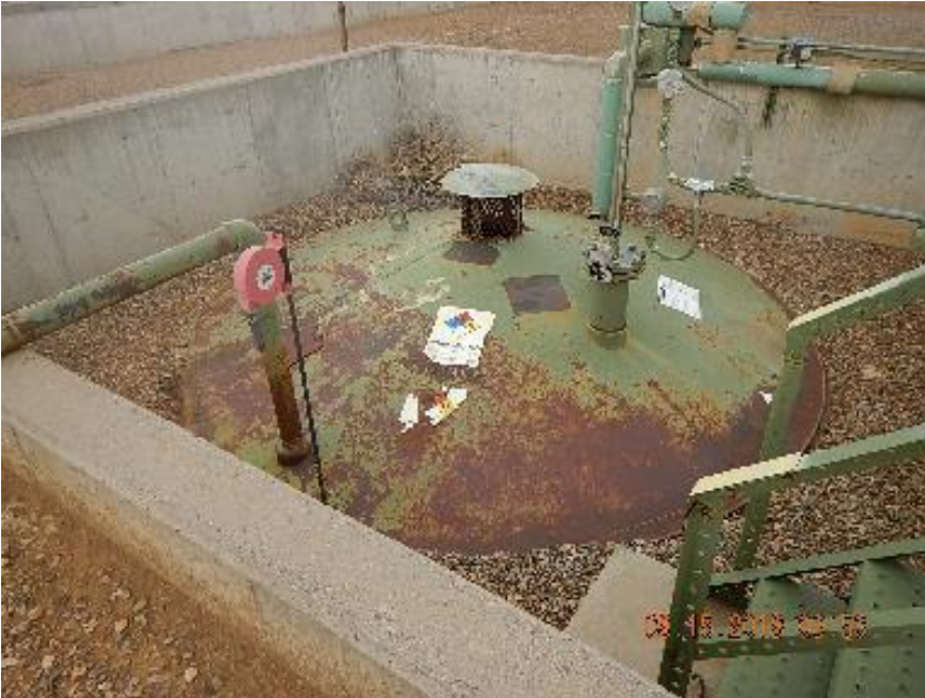
Photo 3: 95 BBL tank peeling tank labels.
