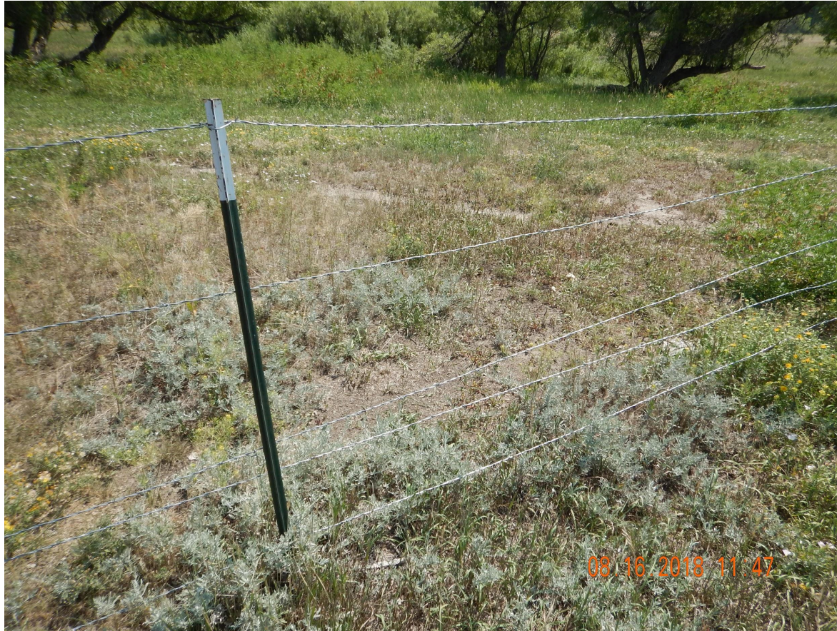
Photo 11. Photo taken from the northeastern perimeter of location on August 16, 2018. Fence repairs are needed to keep cattle out, as the surface owner grazes the adjacent lands.
