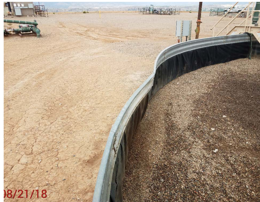
Location Photo #4, damaged containment
