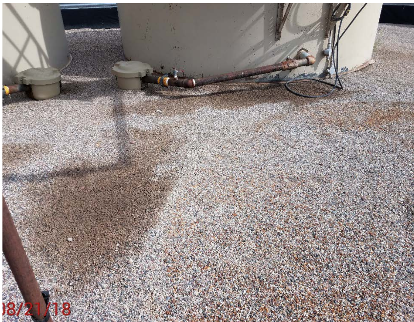
Location Photo #5, Stained material in battery containment.
