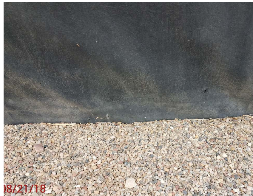
Location Photo #4, holes in secondary liner.
