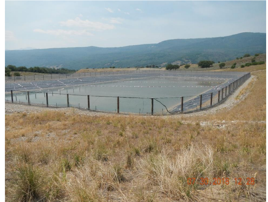
Fence and netting in good condition at Pit Facility ID #454880.
