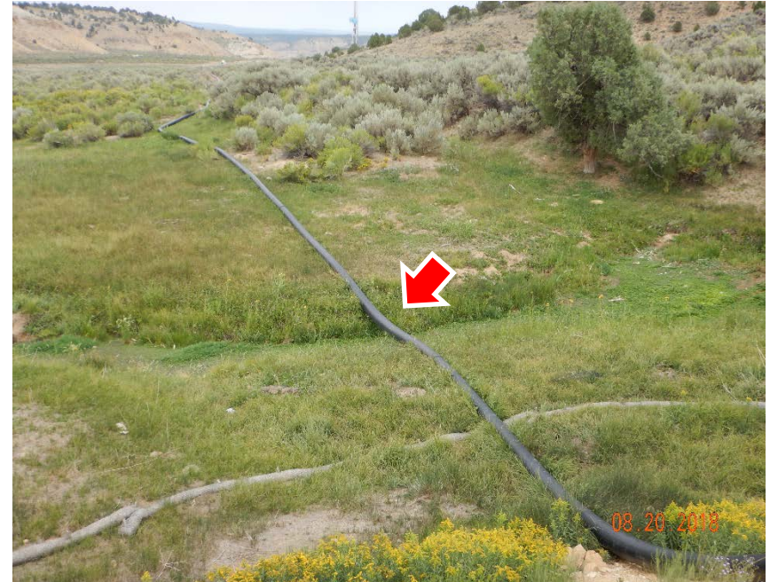
Photo #4 – Looking east along HDPE surface line, which is located at NE corner of location. Red arrow indicates area where line crosses a drainage that acts as a tributary to Black Sulphur Creek.
