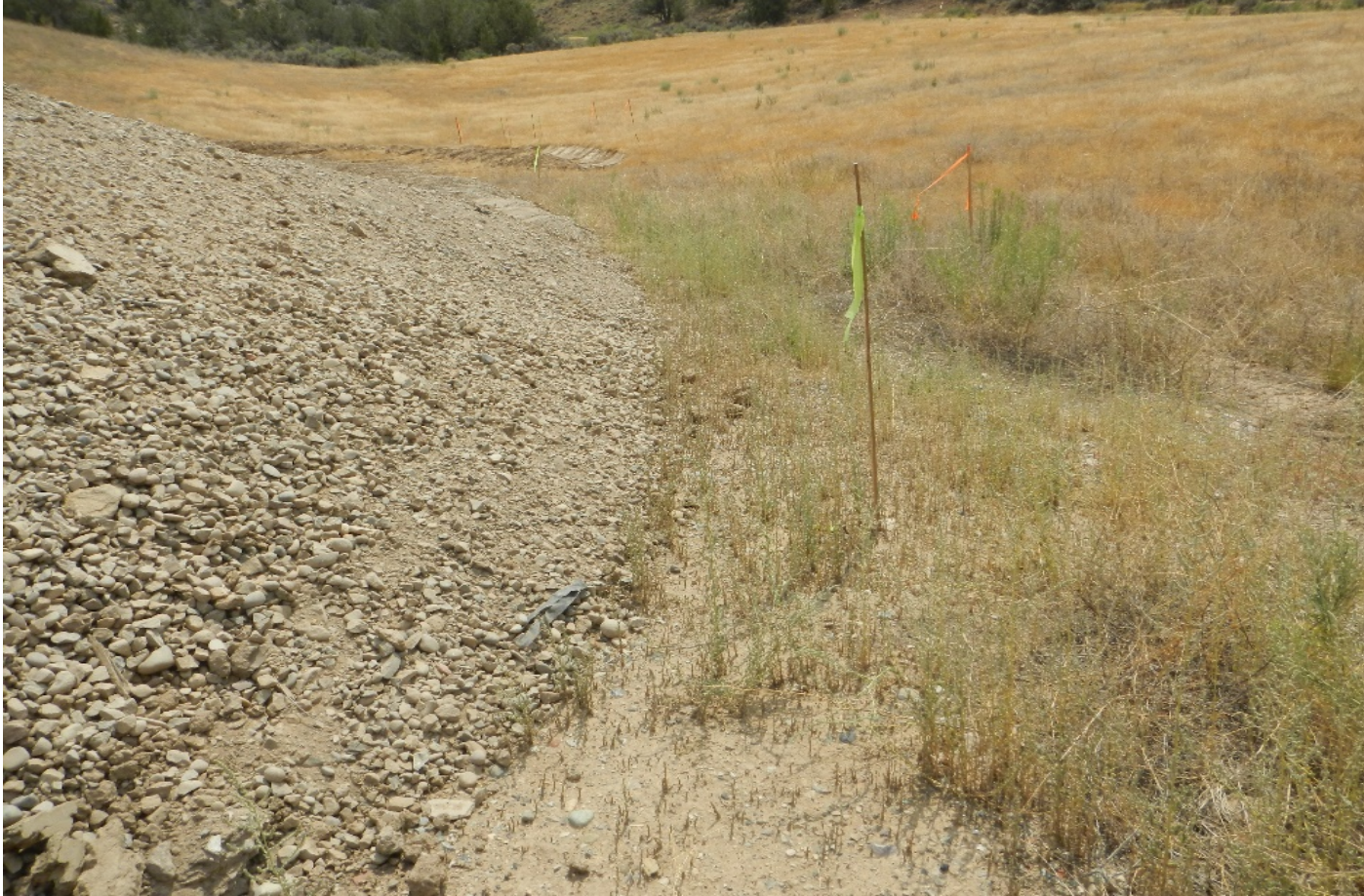
Photo#5: No BMPs installed around Materials Stockpile.
