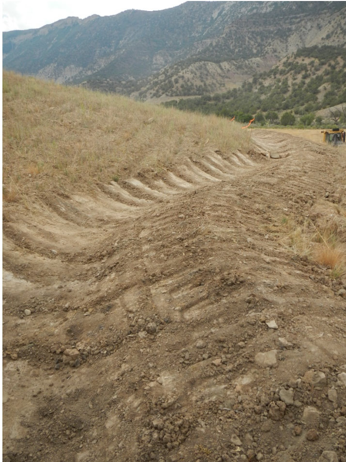
Photo#7: Views of Ditch & Check dams installed at top of Cut Slope.
