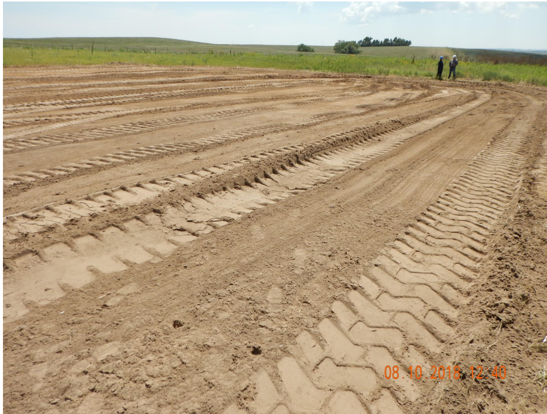
Photo 1. Photo taken from the southwestern location, facing South. Photo illustrates the area that will appear to be used as the sediment basin stormwater area. Operator has installed filter wattles along the entire perimeter of the location during initial construction operations.
