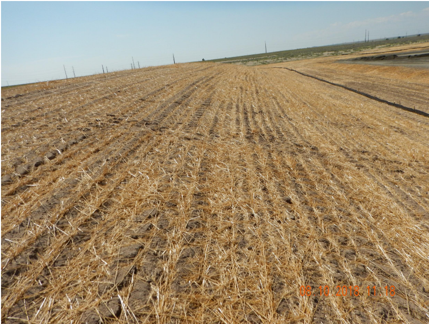
Photo 4. Photo taken from the eastern soil stockpile, facing South. Soil stockpiles have been seeded and crimped with filtrex wattles along the base.
