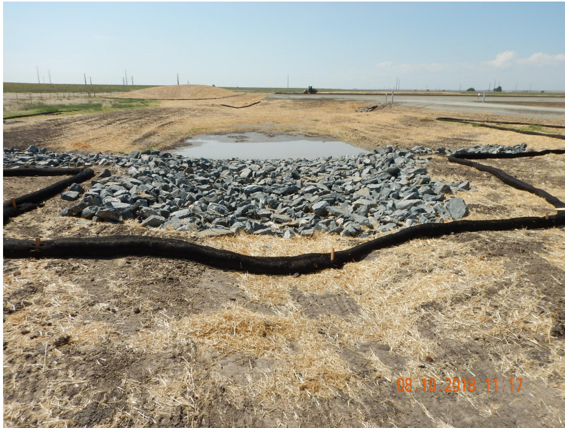
Photo 2. Photo taken from the northeastern perimeter of the location, facing South. Photo illustrates a sediment basin that appears to be in proper functioning condition. Operator has installed a ditch that continues north of the sediment basin. Operator will be responsible for that ditch disturbance (contouring and vegetation standards).
