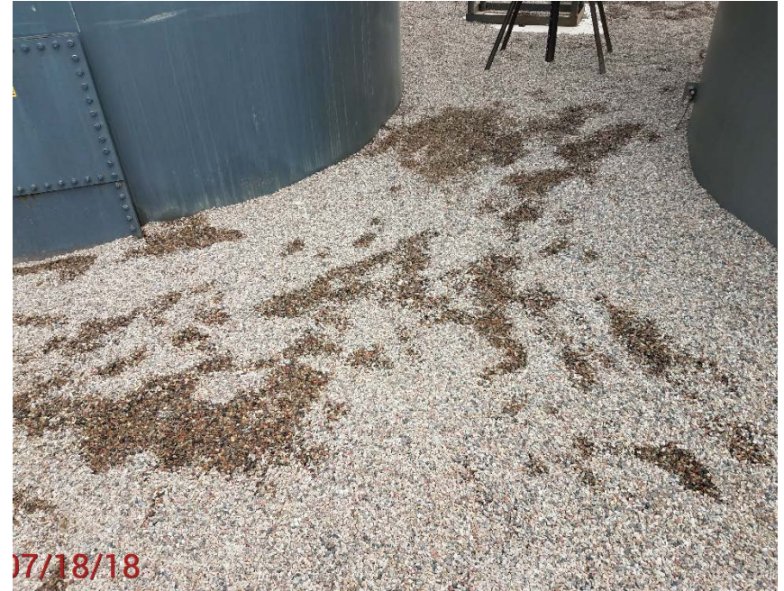
Location Photo # 6, Oil stained material in battery containment
