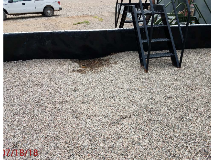
Location Photo #8, Oil stained material in battery containment
