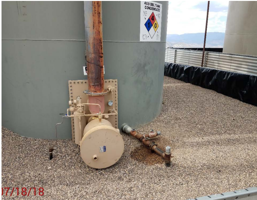
Location Photo #9, Oil stained material in battery containment
