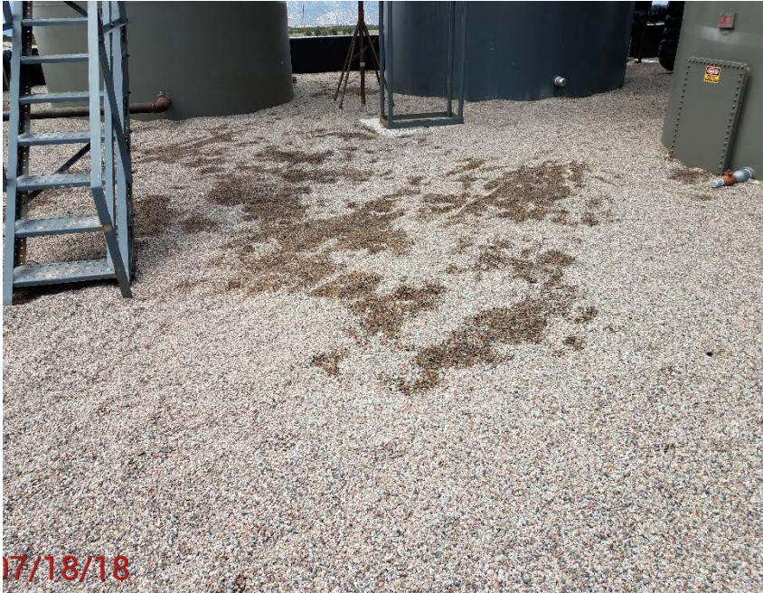
Location Photo # 5, Oil stained material in battery containment
