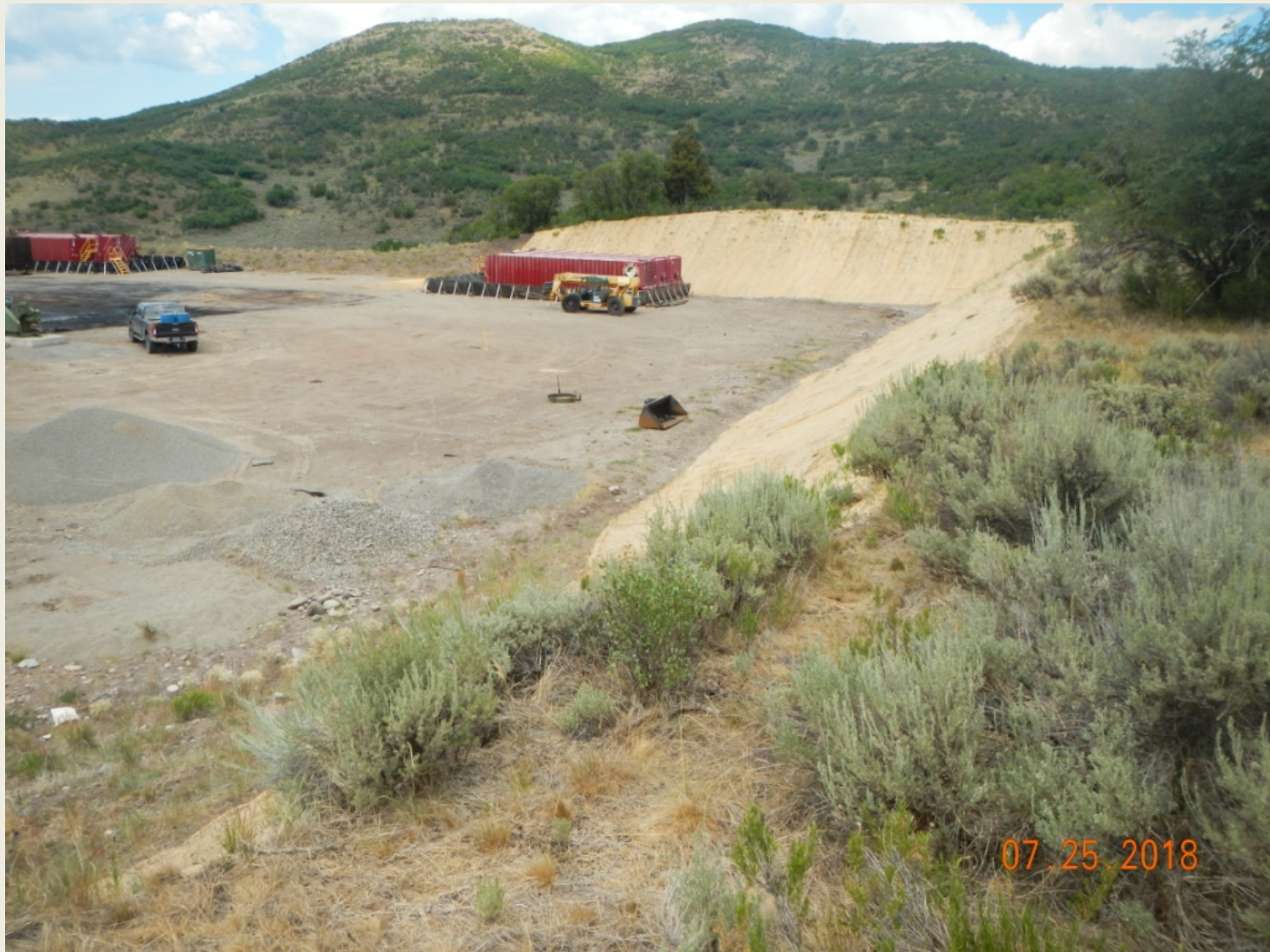
Photo 3. View of the eastern portion of the southeastern corner facing northward. Straw blankets and diversion ditch are in place and appear to be functioning at this time.
