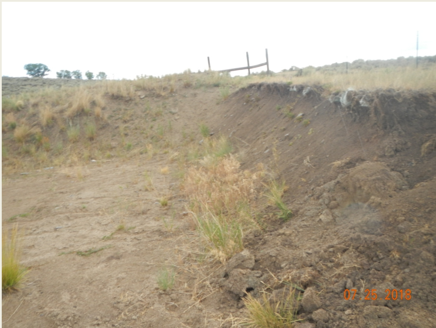
Photo 7. View of cut-slope along northeastern edge of project area that is sloughing and eroding. Erosion controls are needed to stabilize this slope.
