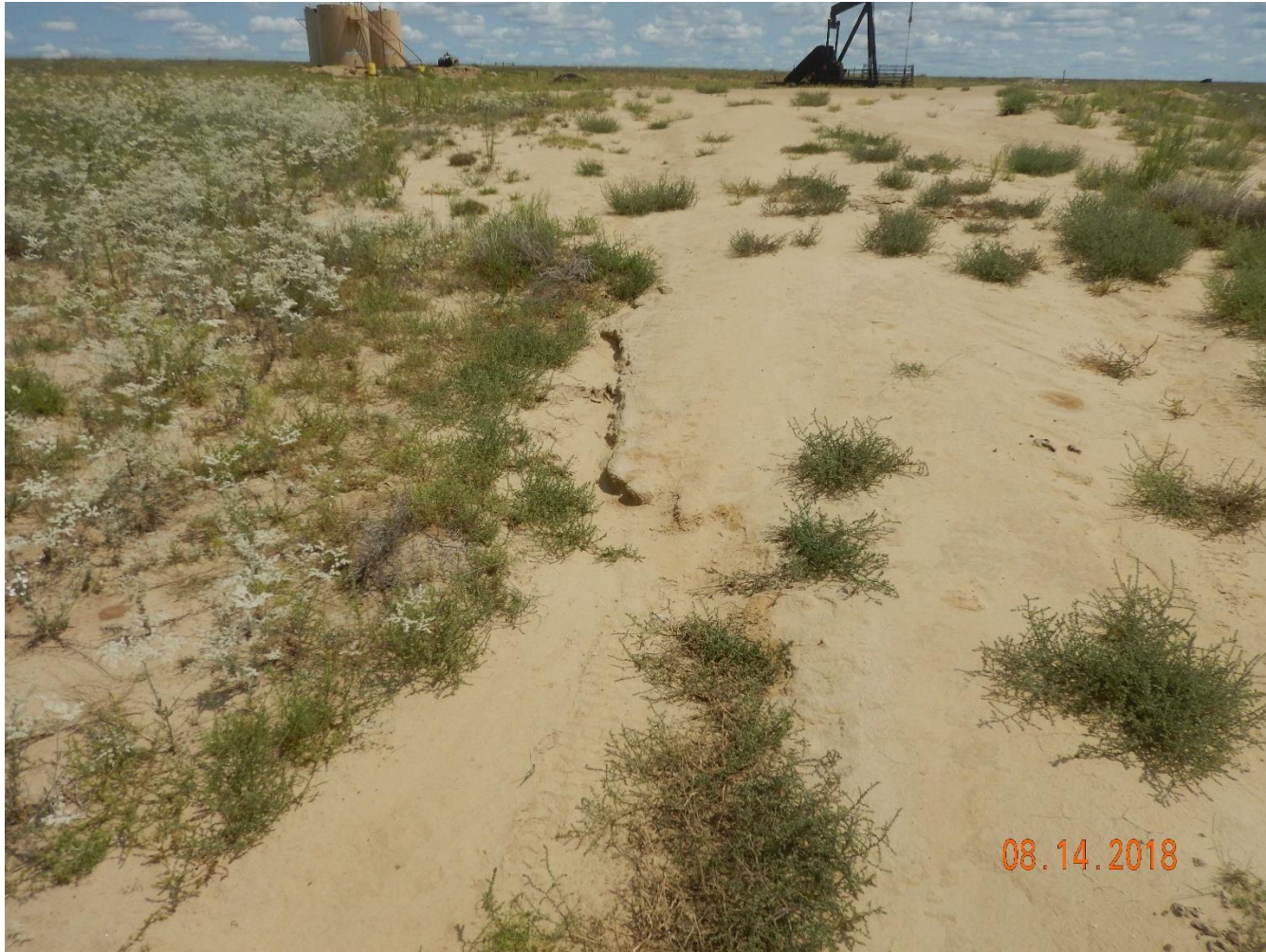
Photo 1: Photo taken from the north end of the location. Photo shows erosion has continued to degrade access road and location. Unable to find evidence of maintenance or evidence that the required BMPs have been installed per 1002.f
