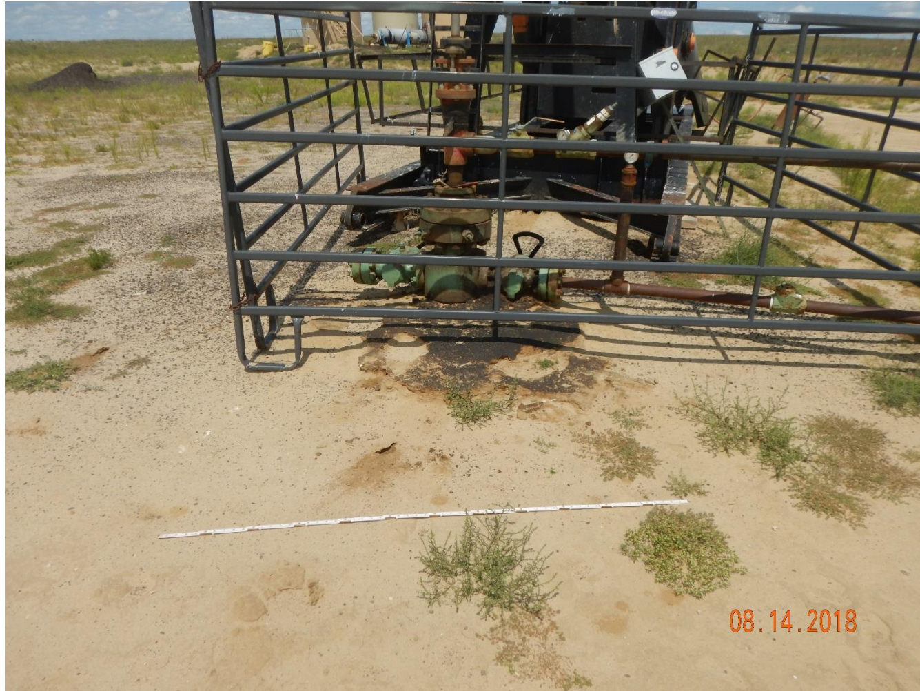
Photo 7: Photo taken from the west end of the well. Previous inspections documented stained soil at wellhead and required operator to remove and/or remediate stained soil. Photo shows soils at wellhead have not been removed, or remediated. Stained soils can also be found in areas surrounding the well. 6 foot measuring stick for reference.
