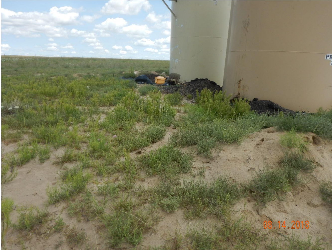
Photo 11: Photo taken from the northwest end of the tanks on location, facing east. Previous inspections documented that the berms around the tanks were inadequate and required operator to repair or install berms, or secondary containment devices. Photo shows berms, or other secondary containment devices have not been repaired or installed; berm missing from the northern end of the tanks. Photo shows additional signage on tanks has not been implemented.
