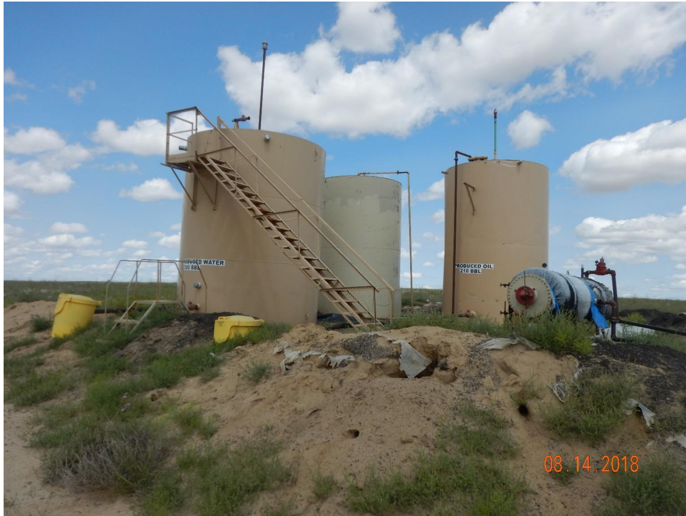
Photo 10: Photo taken from the southwest end of the tanks on location, facing northeast. Previous inspections documented incomplete signage on tanks, including NFPA diamond labeling, and required operator to implement proper signage. Photo shows additional signage has not been implemented.
