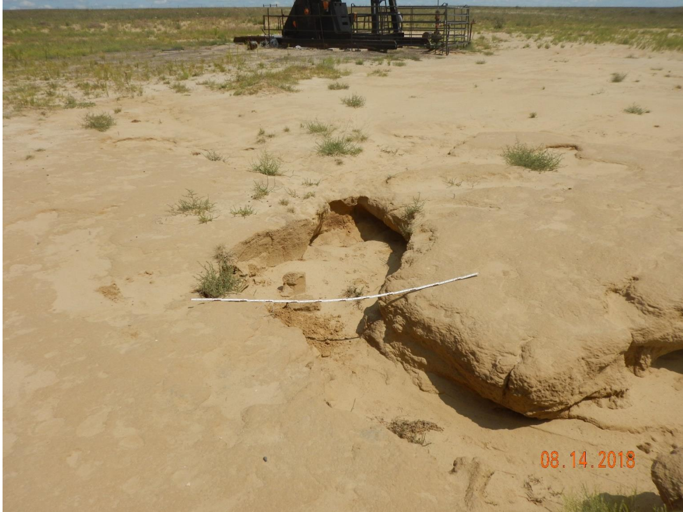
Photo 3: Photo taken from the northwest end of the production area, facing south east. Stormwater erosion has created a large gully on the northwest end of the location (see photos 4-5). Photo shows the “head” of the erosion. Photo shows stormwater erosion has been allowed to continue causing degradation to the location and interim areas. Unable to find evidence of maintenance and stabilization, or evidence that the required BMPs have been installed per 1002.f. 6 foot measuring stick for reference.
