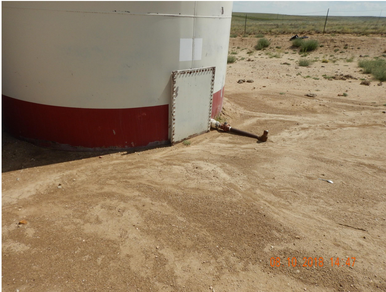
Photo 4. Close up photo taken of the southern tank illustrating sediment erosion accumulation within the containment area and starting to cover valve.
