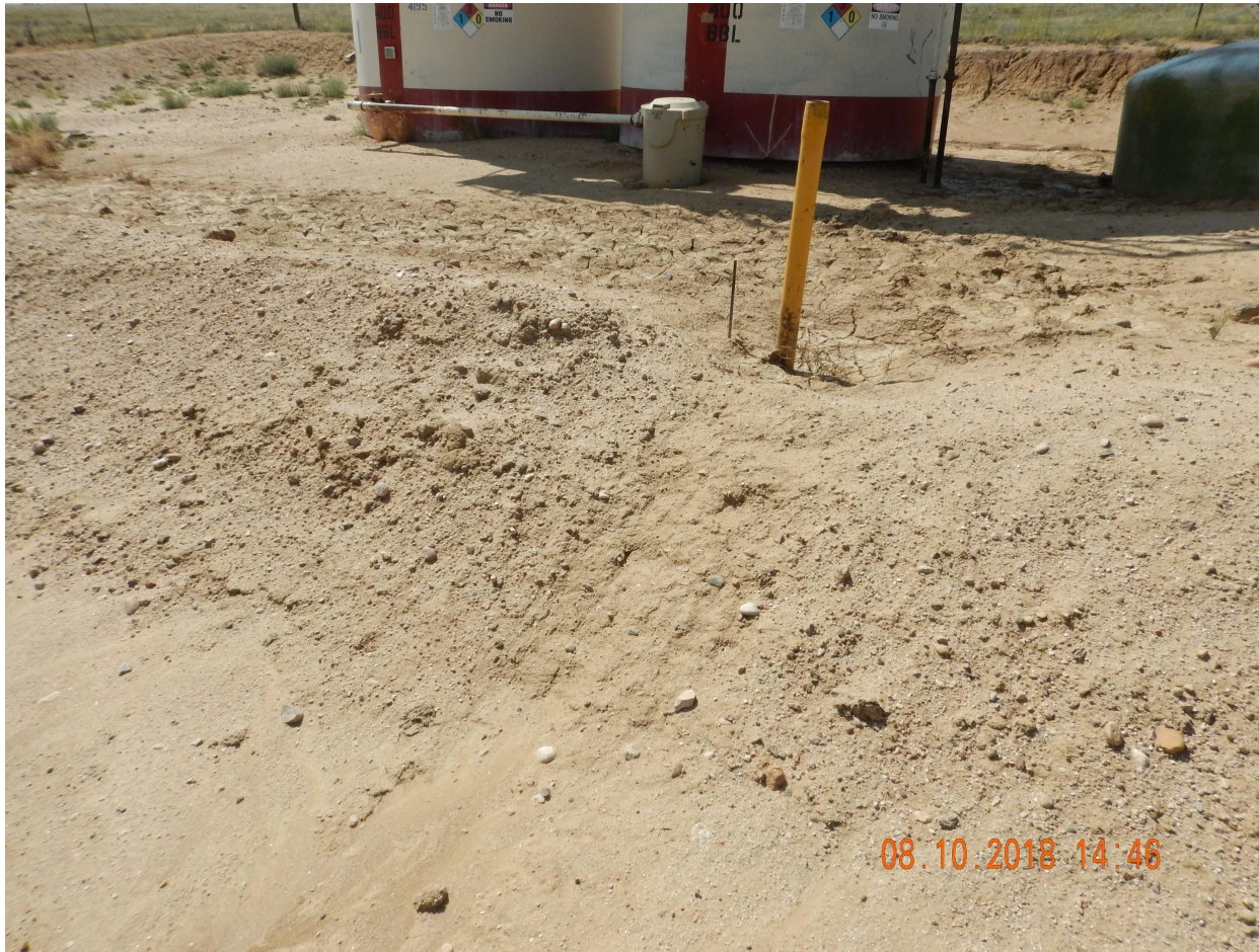
Photo 1. Photo taken from the southern location, facing West. Photo illustrates inadequate berms around tanks. Stormwater has eroded the berm and is eroding underneath one of the tanks- see next photo for a close up.
