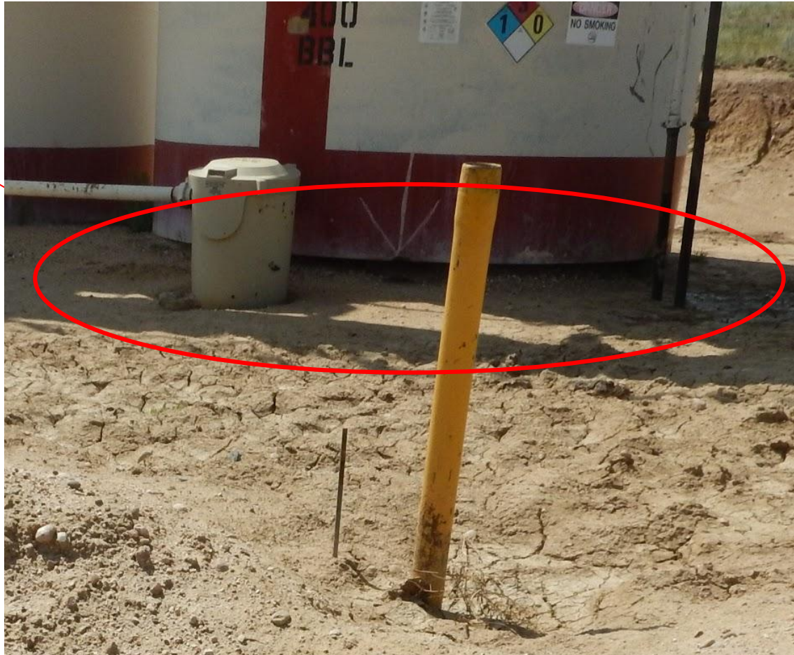
Photo 2. Close up photo illustrating stormwater eroding underneath the tank.
