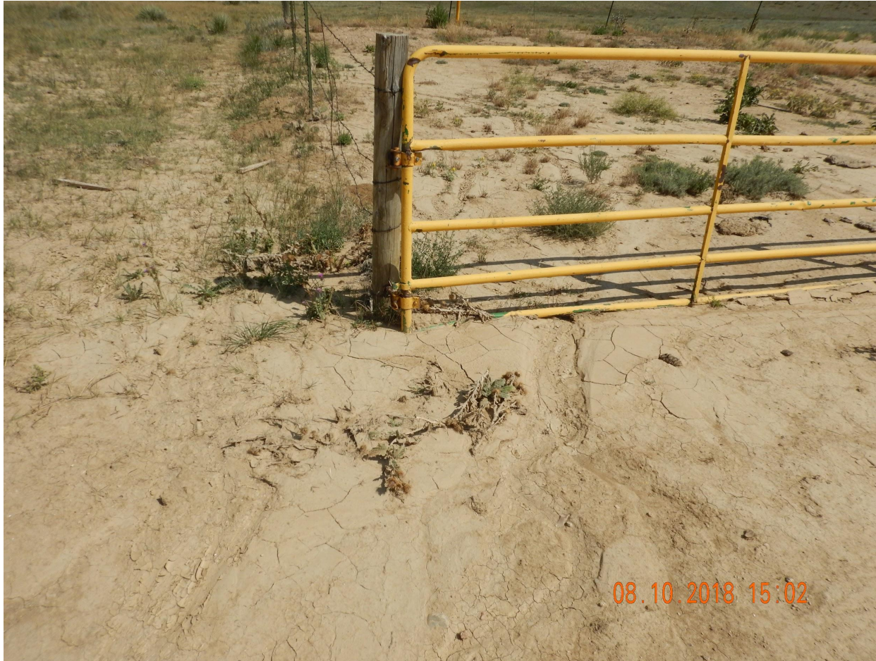
Photo 9. Photo taken from the entrance of the location, facing East. Photo illustrates sediment accumulation from erosion washing downslope cover portions of the gate.
