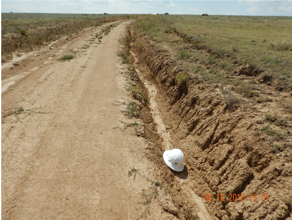
Photo 8. Photo taken along a portion of the access road, facing West. Stormwater erosion is channelizing along portions of the access road and beginning to form gully erosion. In addition, List B Colorado Noxious weeds were observed along portions of the access road.
