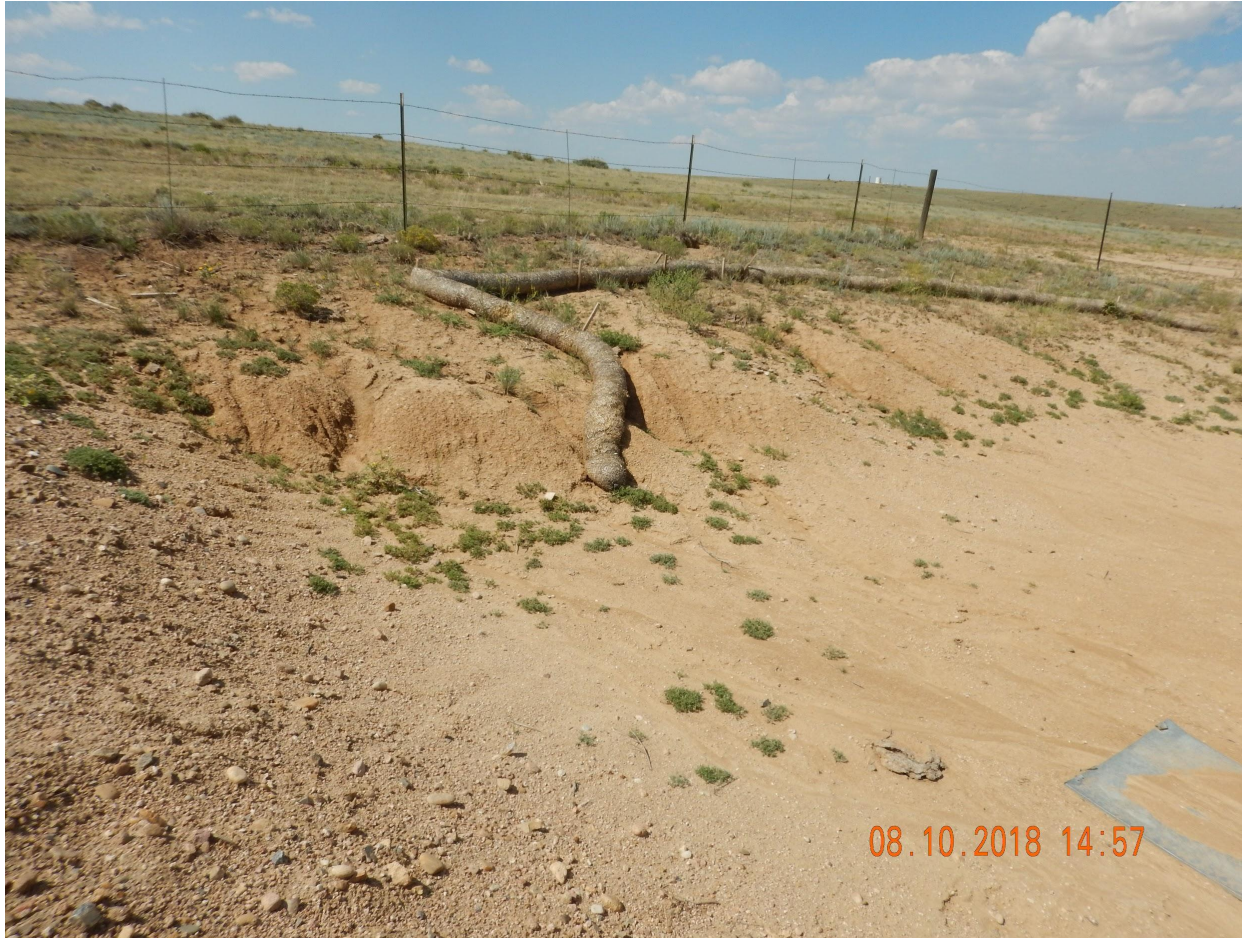
Photo 6. Photo taken of the western cut slope, facing West. Operator has failed to maintain the location to reasonably control and minimize erosion, alteration of natural features and removal of surface materials. Previous inspections required the Operator to repair the rill erosion and stabilize the cut slope. Operator has failed to perform those corrective actions. Also, previous inspections noted the Operator did not properly install wattle BMPs, as this photo illustrates.
