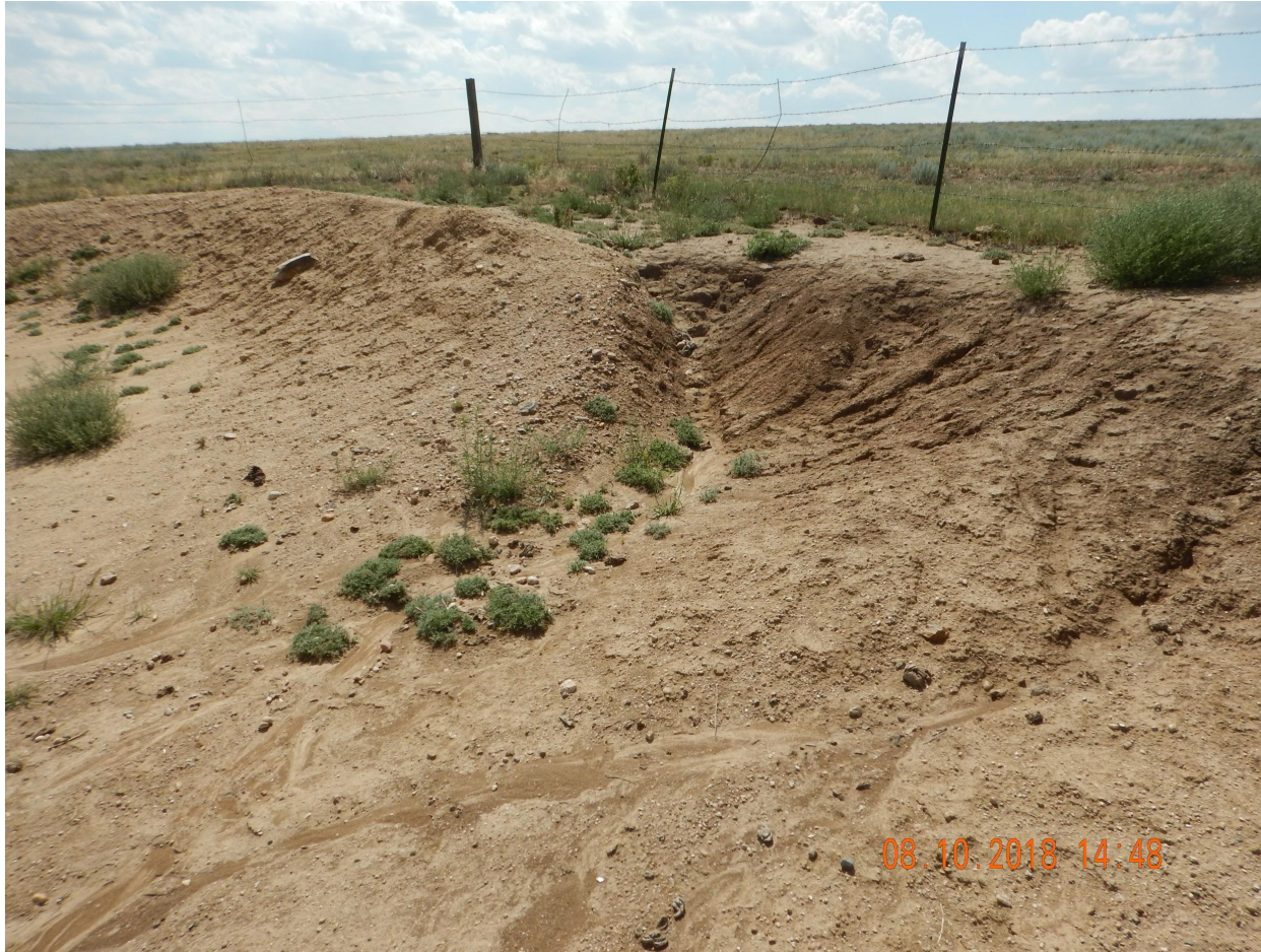
Photo 5. Photo taken of the southwestern tank battery berm, facing South. Stormwater has eroded the berm and sediment filling the containment area.
