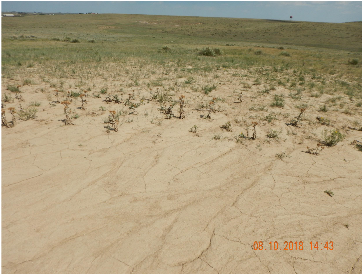
Photo 10. Photo taken from the second discharge point off the access road, facing East. Photo illustrates sediment discharging into the adjacent land with no stormwater control BMP.
