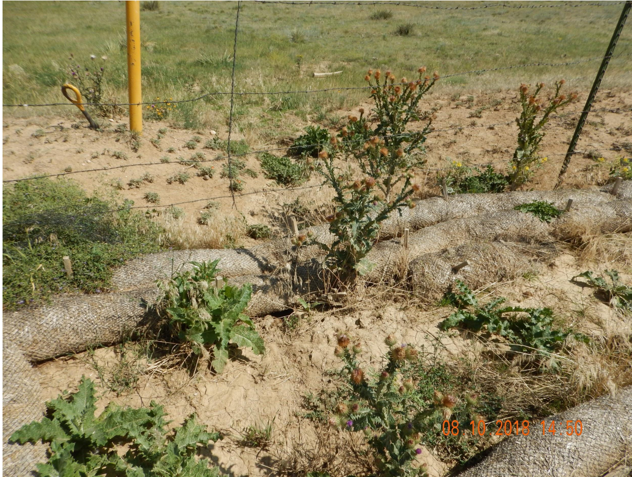
Photo 7. Photo taken from the southeastern location, facing East. Stormwater is eroding underneath the wattle BMPs, as this is one of the observed sediment discharge points off location. BMPs are inadequate which was mentioned in previous inspections. Photo also illustrates List B Colorado Noxious weeds. Four of the five List B Colorado noxious thistles were observed throughout the location and access road.
