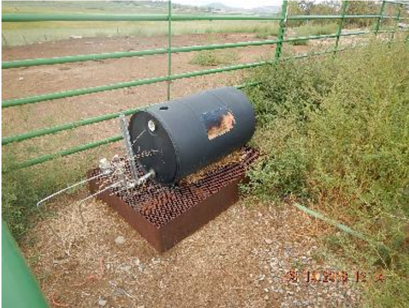
Photo 3: Unreadable chemical tank label and missing filler cap at the Argenta 18.
