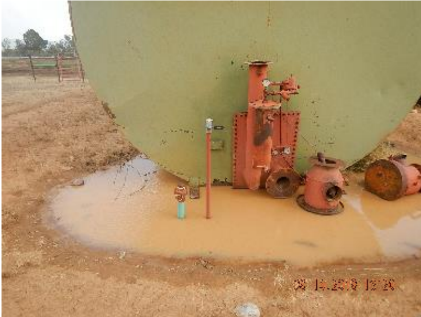
Photo 11: Disconnected risers at back of production tank.
