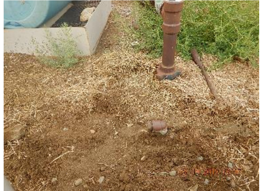
Photo 12: Unused 1" steel riser at Argenta 19 wellhead.
