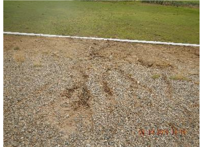
Photo 2: Erosion channels on the E fill slope.
