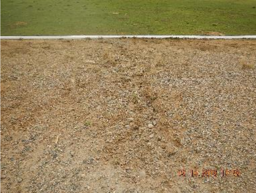
Photo 3: Erosion channel on the E fill slope.
