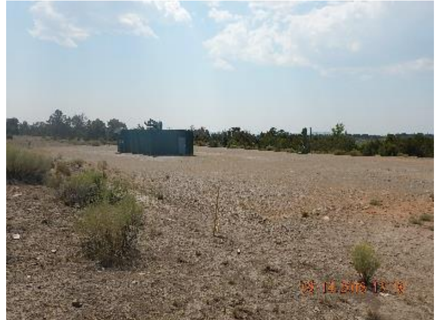
Photo 16: Location overview current inspection.
