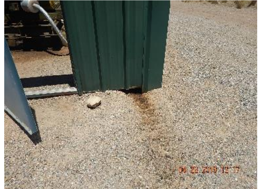
Photo 6: Impacted soil and gravel at exhaust outlet from previous inspection.
