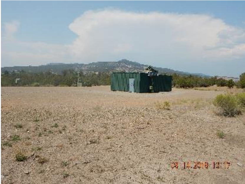
Photo 15: Location overview current inspection.
