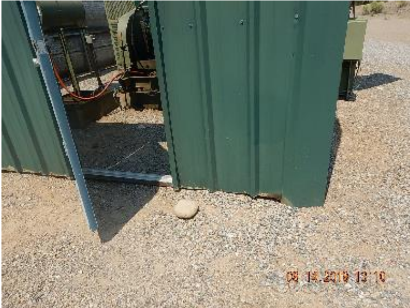
Photo 5: Cleaned up area at old exhaust outlet.
