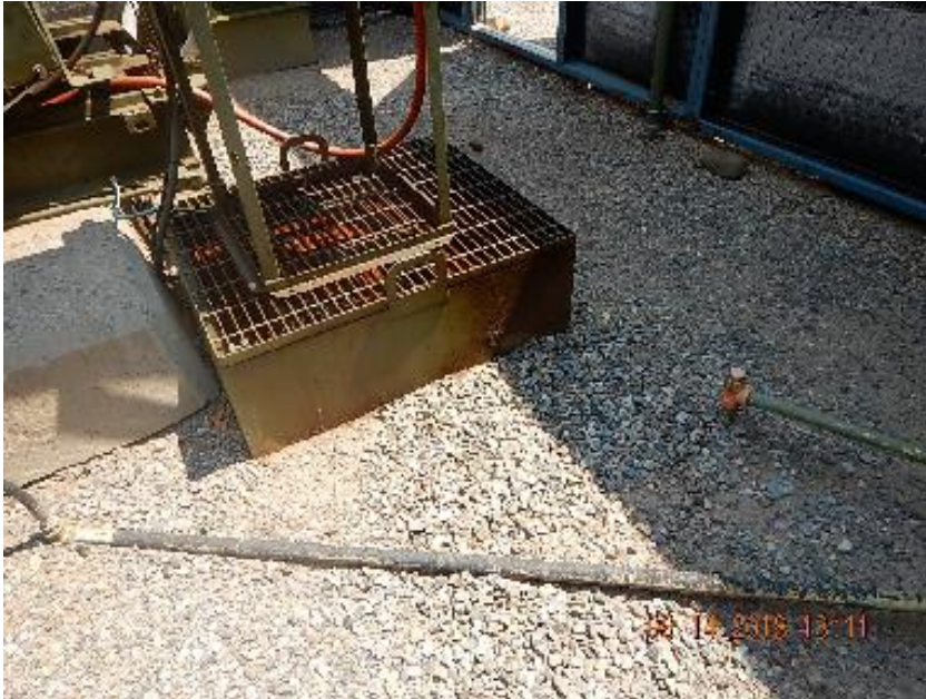
Photo 7: Cleaned up area at lube oil tank.
