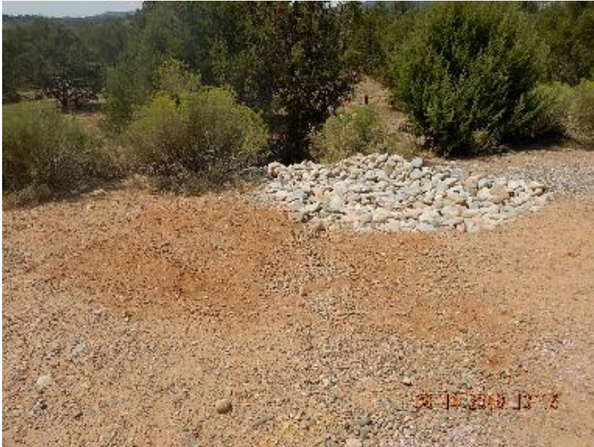
Photo 9: Repaired erosion channel.
