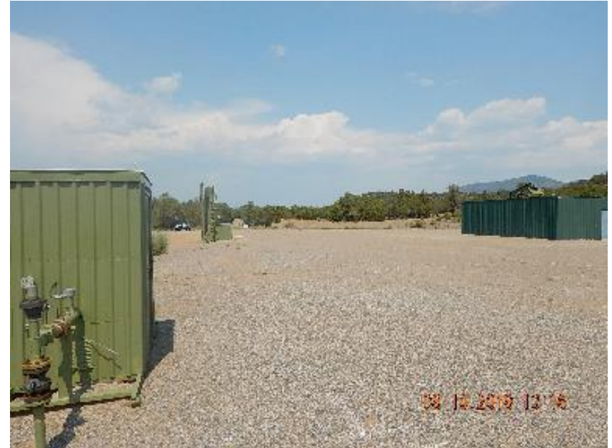
Photo 14: Location overview current inspection.
