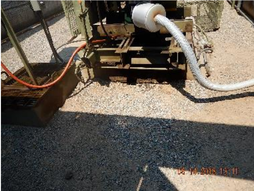
Photo 3: Cleaned up area at rear of pump jack.
