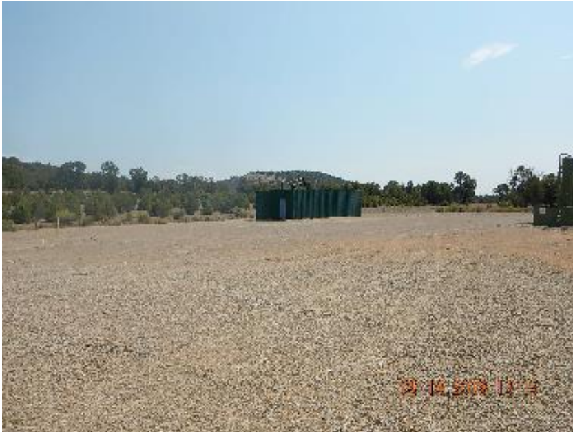
Photo 13: Location overview current inspection.
