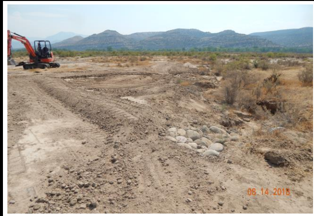
Erosion Repair & Berm Installation on the West Side of the Pad
