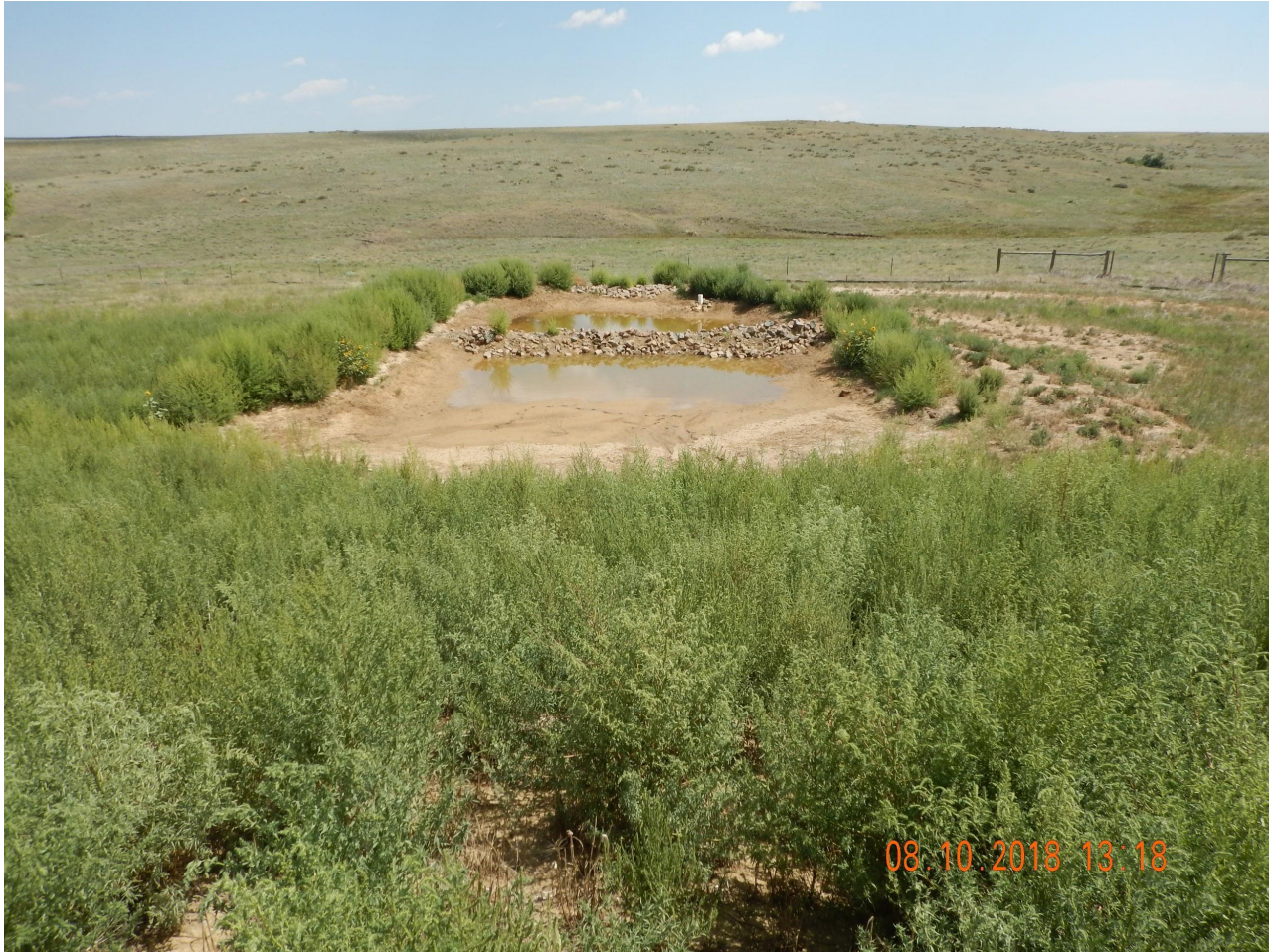
Photo 3. Photo taken from the eastern perimeter of the location, facing East. Sediment basin appears to be properly functioning. No sediment discharge was observed off location.
