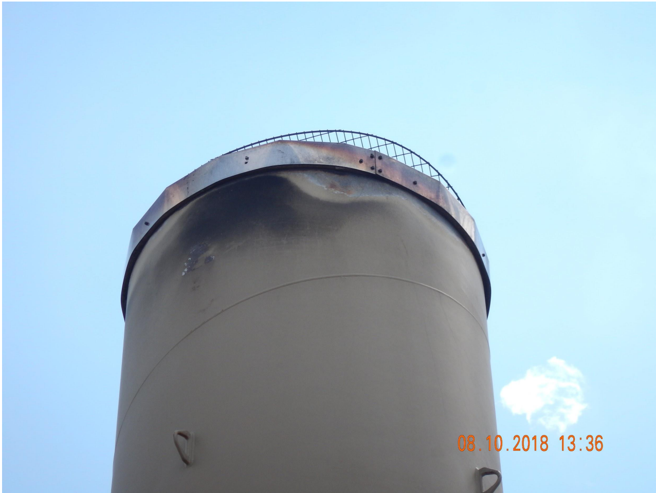
Photo 6. Photo taken from the eastern production area. Wildlife screen does not appear to be centered. Operator shall comply with Rule 605.b.(7).
