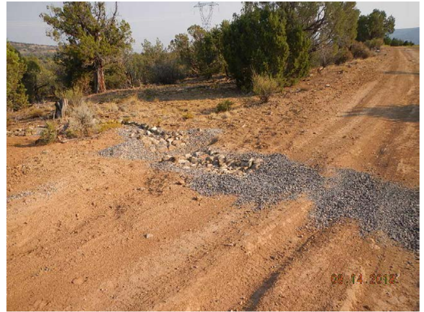
Photo 2. Sediment trap added.
