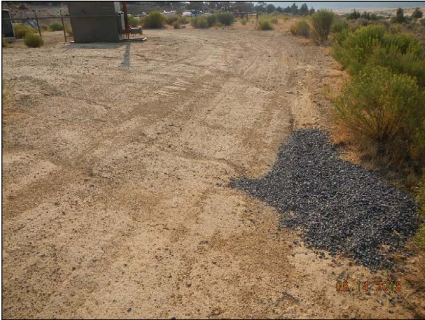
Photo 1. Gravel added to area of erosion and sediment migration. Continued monitoring will be necessary to determine if it is effective.
