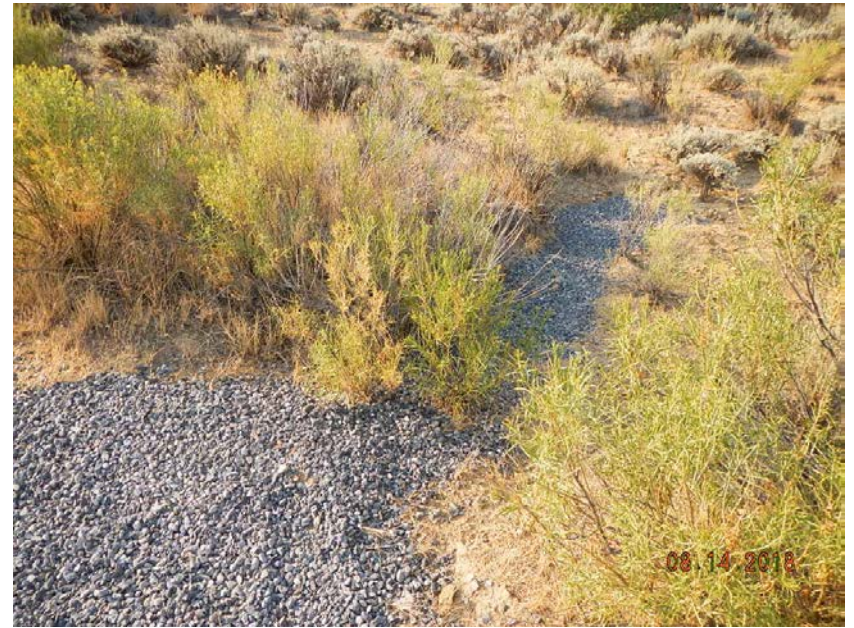
Photo 2. Gravel added to area of erosion and sediment migration. Continued monitoring will be necessary to determine if it is effective.
