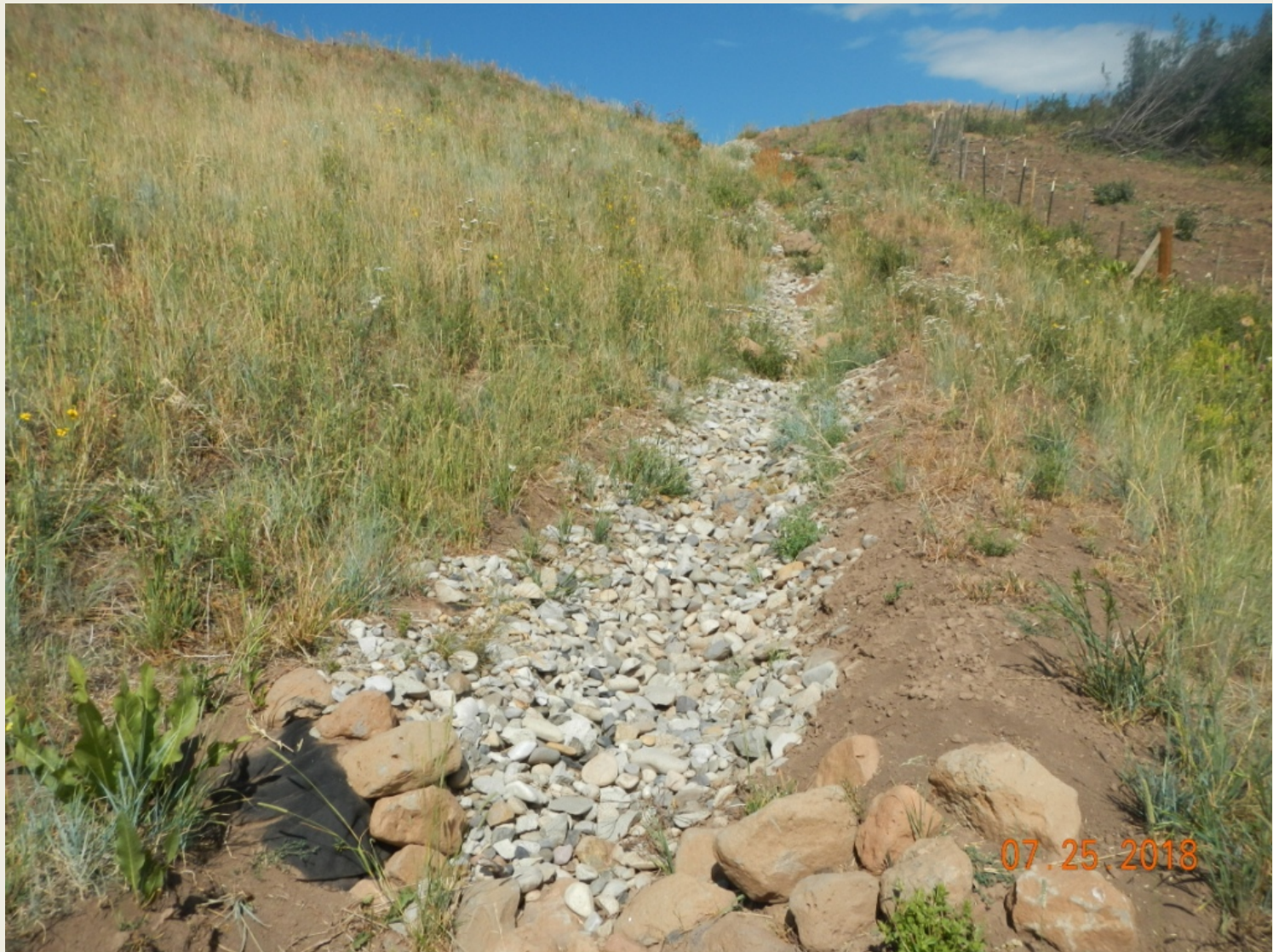
Photo 6. View of the northeastern portion of the project area rock run-down appears to be functioning.
