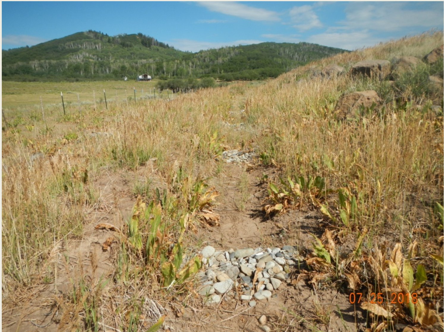
Photo 2. View of the southwestern portion of the project area from the southern corner facing northwestward. Rock check dams appear to be functioning. Vegetation is becoming established on fill slopes with grasses, shrubs, and forbs such as smooth brome ( Bromus inermis ), snowberry ( Symphoricarpos albus ), and mules ears ( Wyethia sp.).
