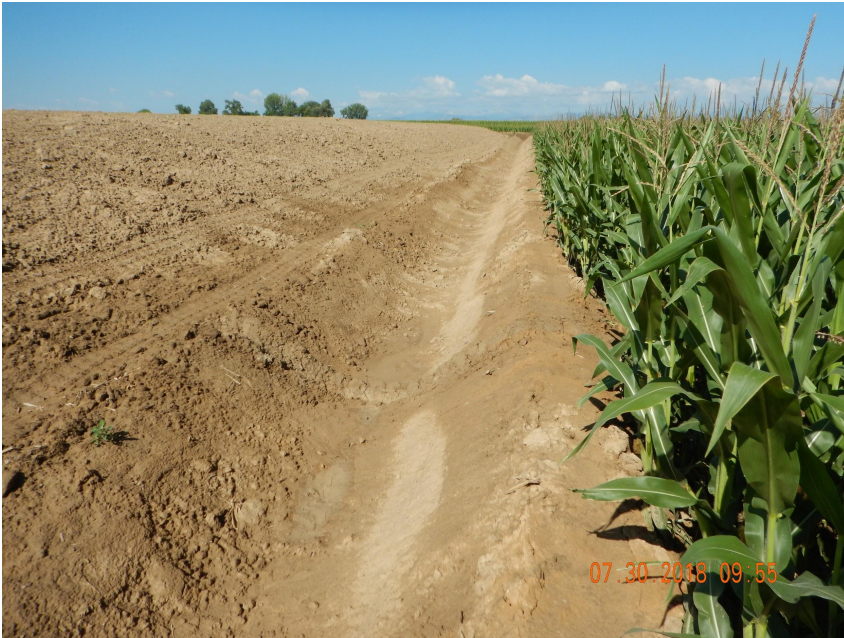
Photo 7. Photo taken from the northern perimeter of the location, facing West. Photo illustrates a ditch and berm BMP and the topsoil stockpile.
