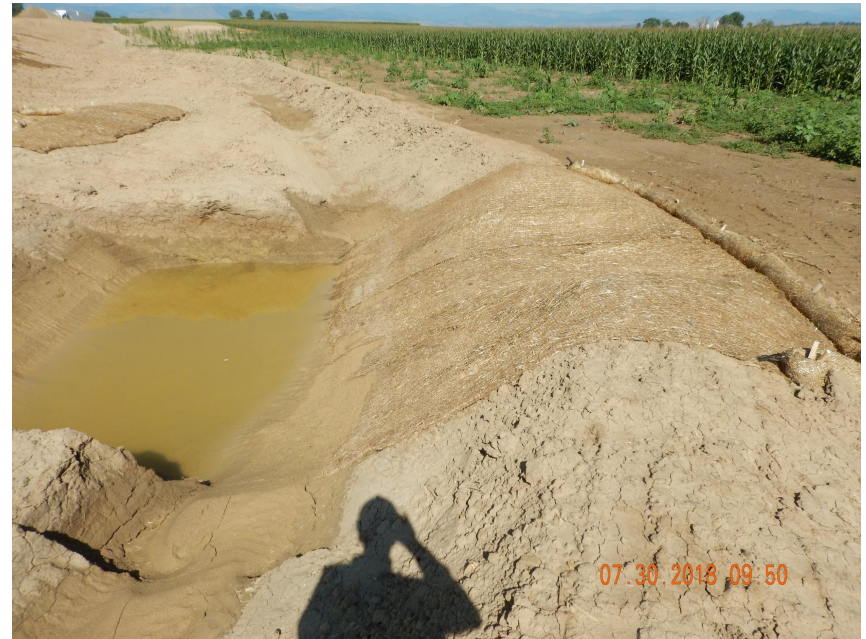
Photo 4. Photo taken from the outlet area of the northeast sediment trap, facing West. No sediment discharge was observed. Operator also has a retention area, not shown in this photo, upslope from this sediment trap.
