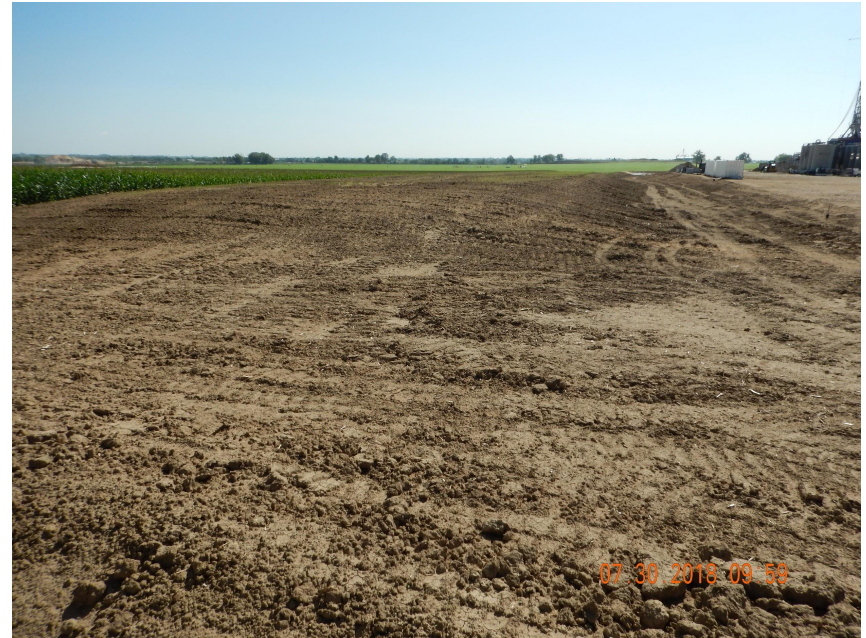
Photo 8. Photo taken from the northwestern perimeter of the location, facing East. Topsoil stockpile has been stabilized with equipment tracking and appears to be seeded. Germination was observed along portions of the topsoil stockpile.
