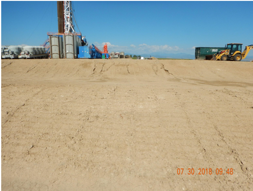
Photo 3. Photo taken of the eastern fill slope, facing West. Photo illustrates rill erosion. Operator shall stabilize fill slopes to minimize site degradation.
