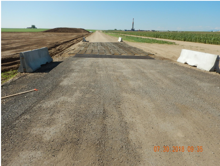
Photo 1. Photo taken from the entrance of location off CR 20.5, facing South. Operator has installed tracking device BMPs and appears to be in proper functioning condition.
