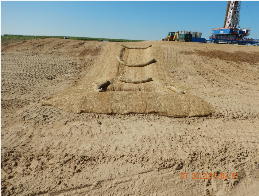
Photo 5. Photo taken from the northeast perimeter of the location, facing South. Photo illustrates a stabilized outfall from the retention pond which is directed to the sediment trap previously shown in Photo 4.
