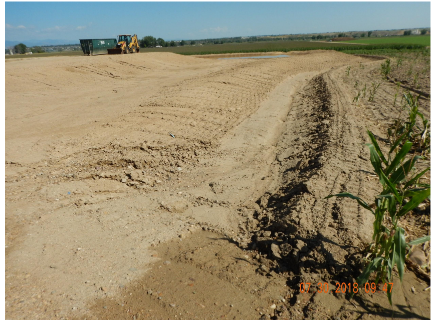
Photo 2. Photo taken from the entrance of location, facing North. Ditch and berm BMP has been installed around the entire perimeter of the location.
