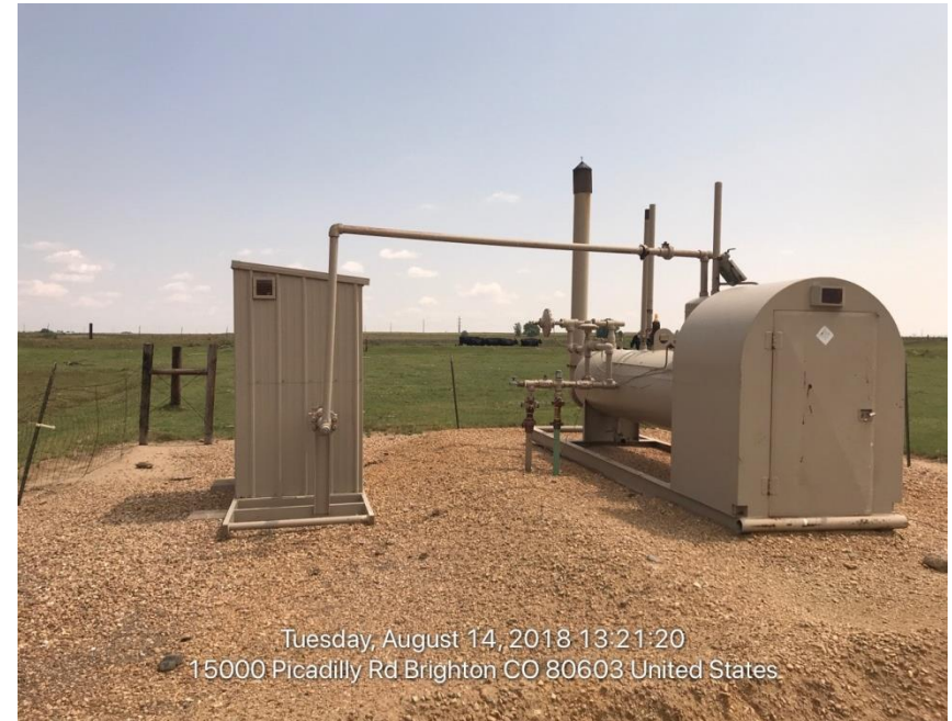
Photo#2 Gas Meter and Separator
