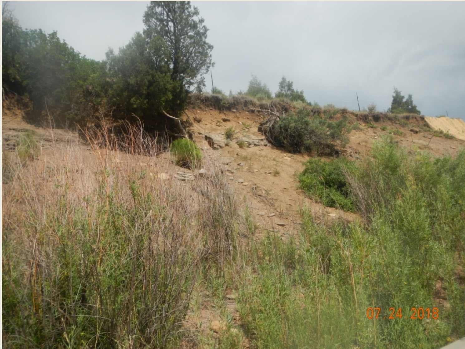
Photo 5. Another view of northeastern cut-slope showing areas that are not stabilized. Trees on the slope have either fallen or have exposed roots from erosion. Additional stabilization measures are needed to stabilize these areas, especially at the top of the slope.
