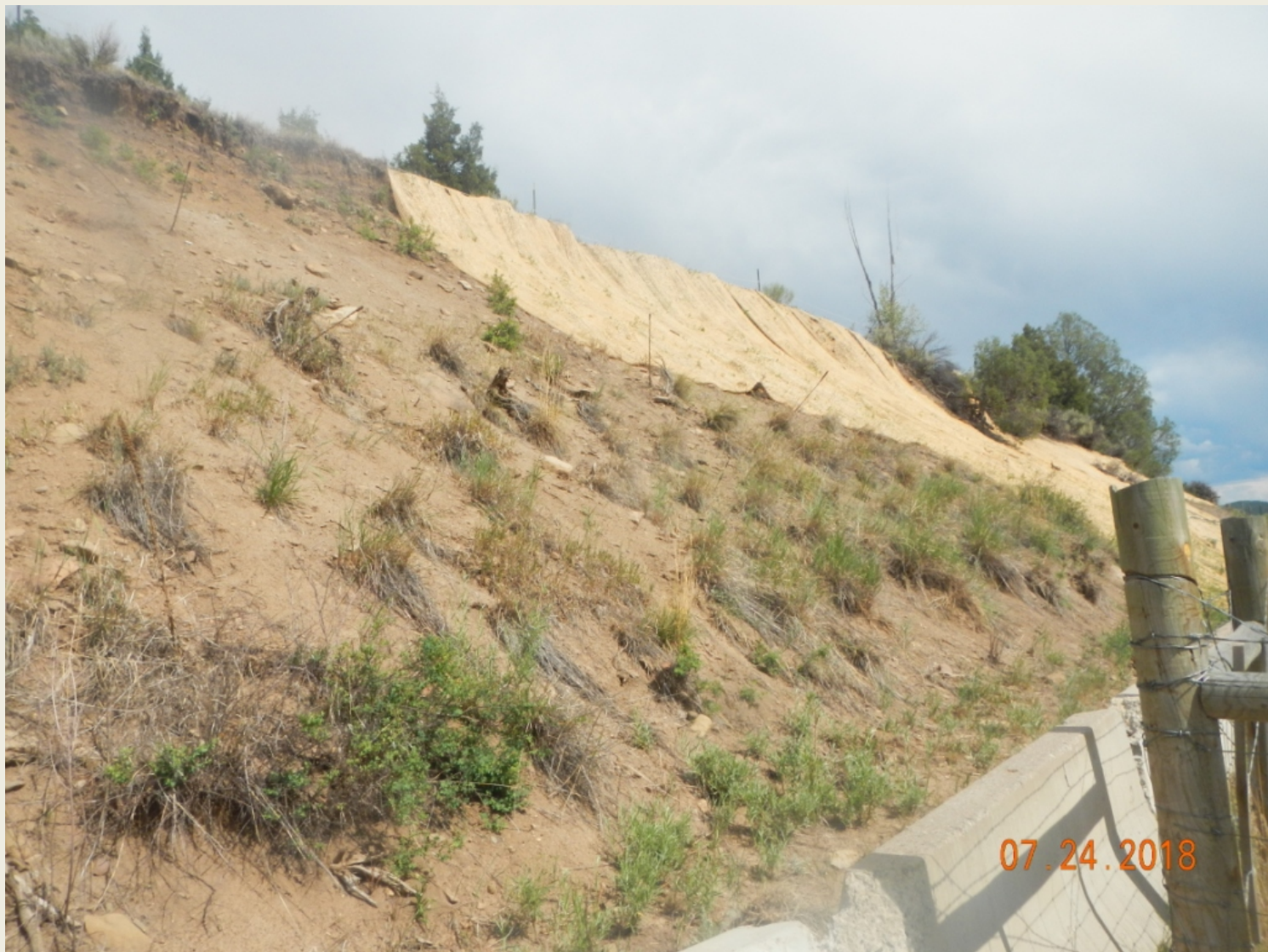
Photo 4. View of the northeastern cut-slope showing areas that are not stabilized with jute mat.
