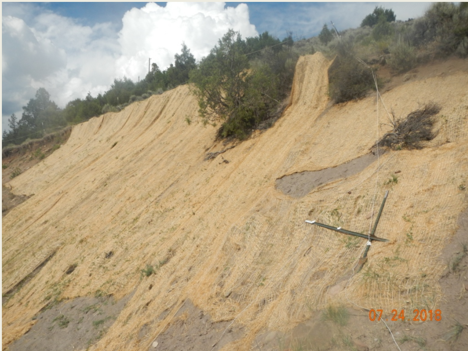
Photo 2. Another view of cut-slope with recently installed blanket. Portions of blanket are torn and insufficiently anchored.
