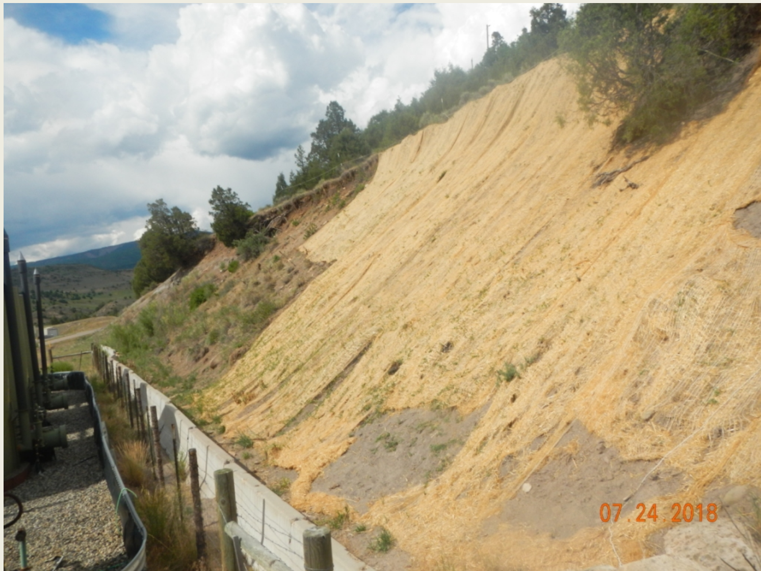
Photo 1. View of the eastern cut-slope from the southeastern corner facing northward. Erosional blanket is installed.
