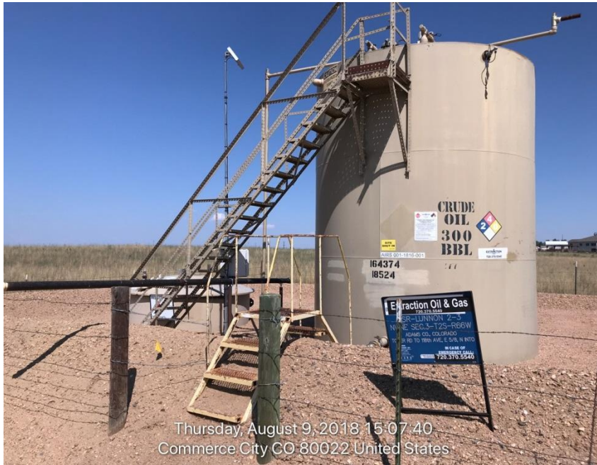
Photo#1Production tank and produced water pit
