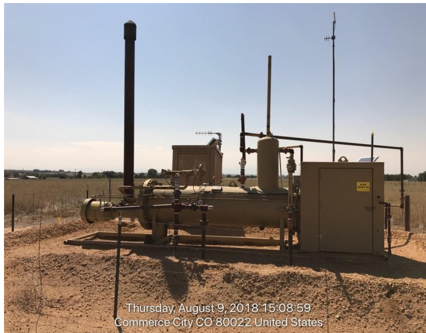
Photo#3Separator and Gas Meter
