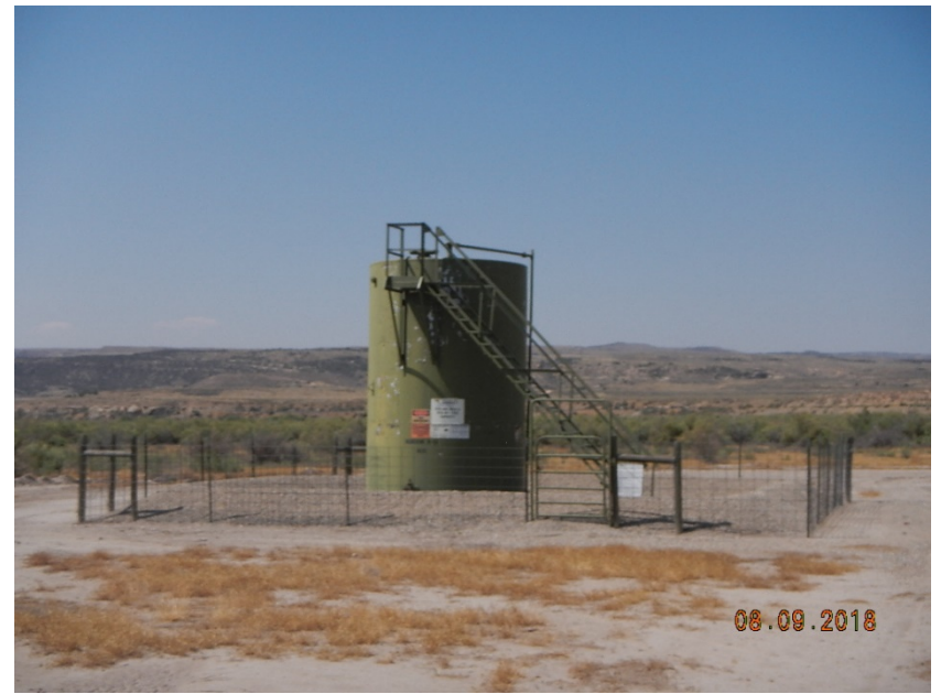
Photo 2. Tank in earth containment.
