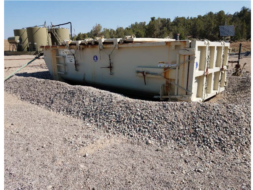
Location Photo #2, Secondary berm around tank installed. Sign was updated.
