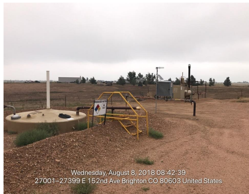
Photo#3 Water Pit/Gas Meter and Separator
