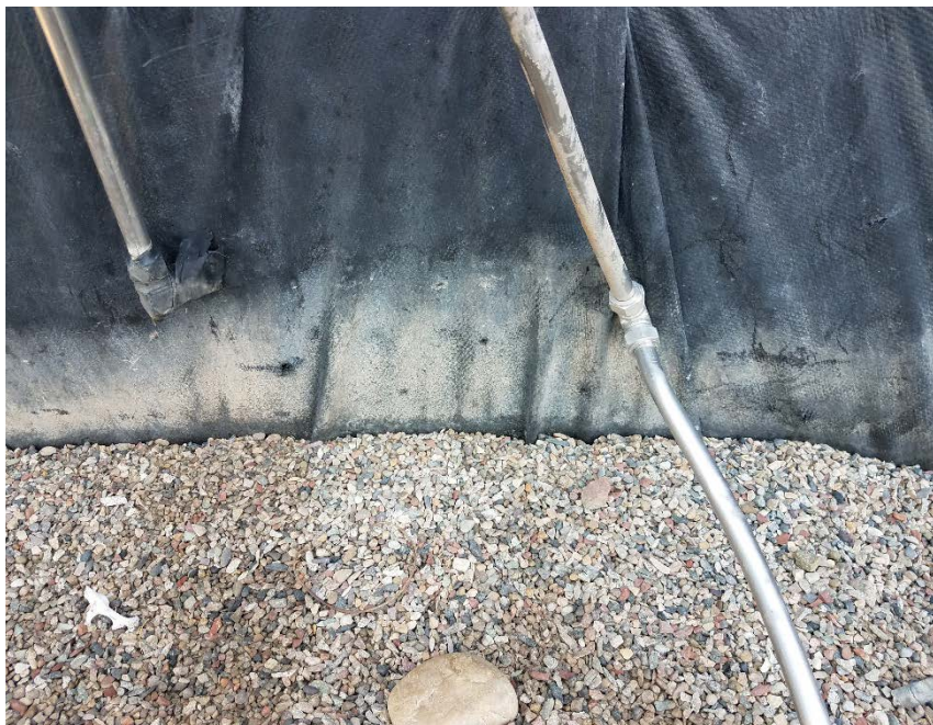
Location Photo #7, Holes in secondary containment liner.
