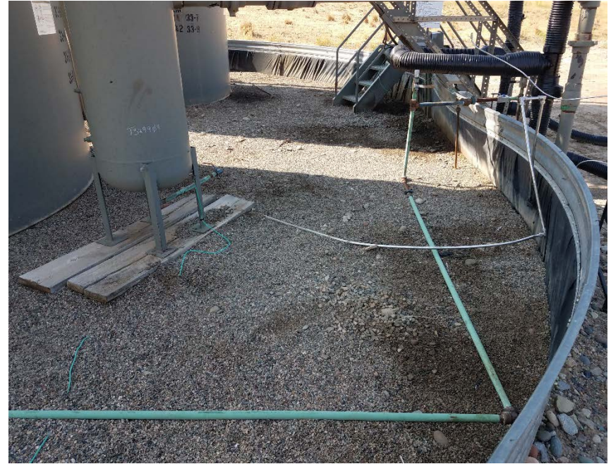
Location Photo #6, Stained rock in tank containment.
