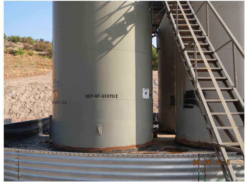
Photo 2. Out of service tank in containment.
