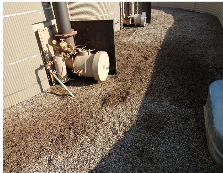
Location Photo #10, Stained rock in battery containment.
