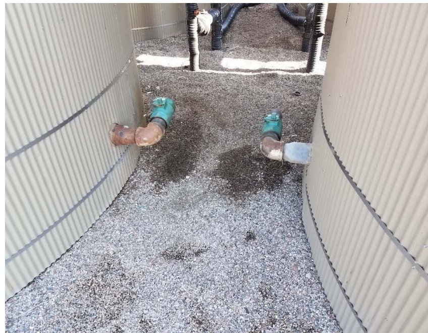
Location Photo #8, Stained rock in battery containment.
