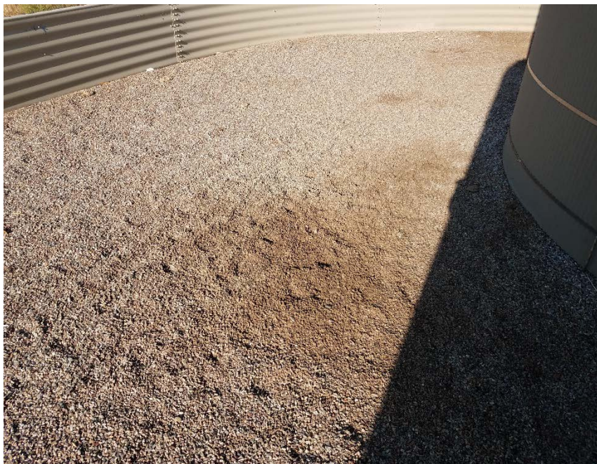
Location Photo #9, Stained rock in battery containment.
