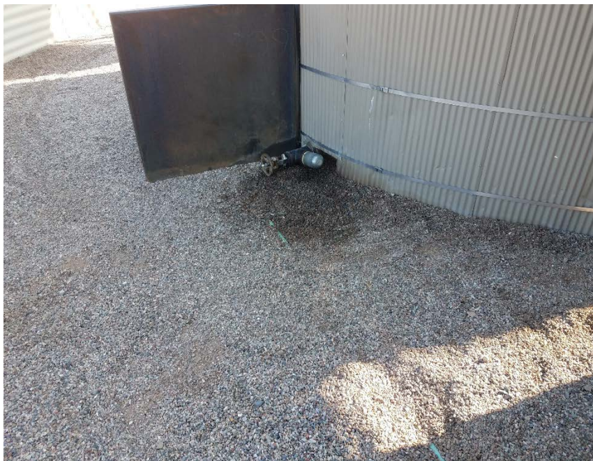
Location Photo #7, Stained rock in battery containment.
