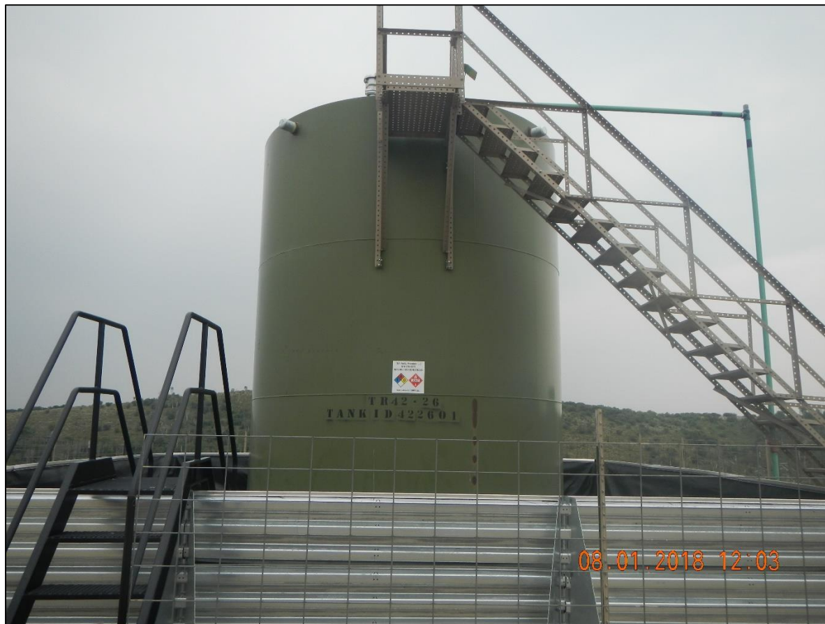
Label has been installed on tank.
