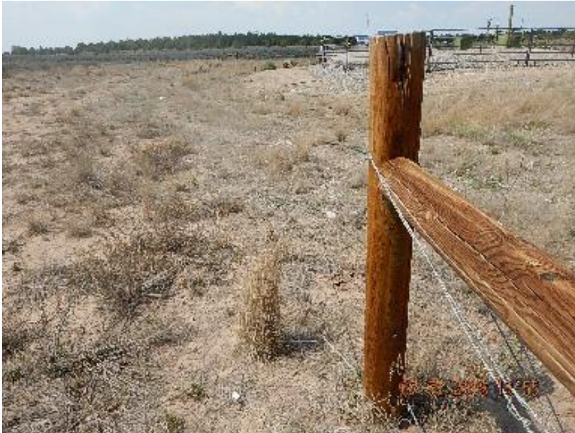
Photo 3: Downed fencing along location perimeter.
