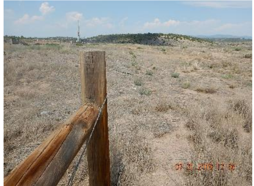
Photo 4: Downed fencing along location perimeter.
