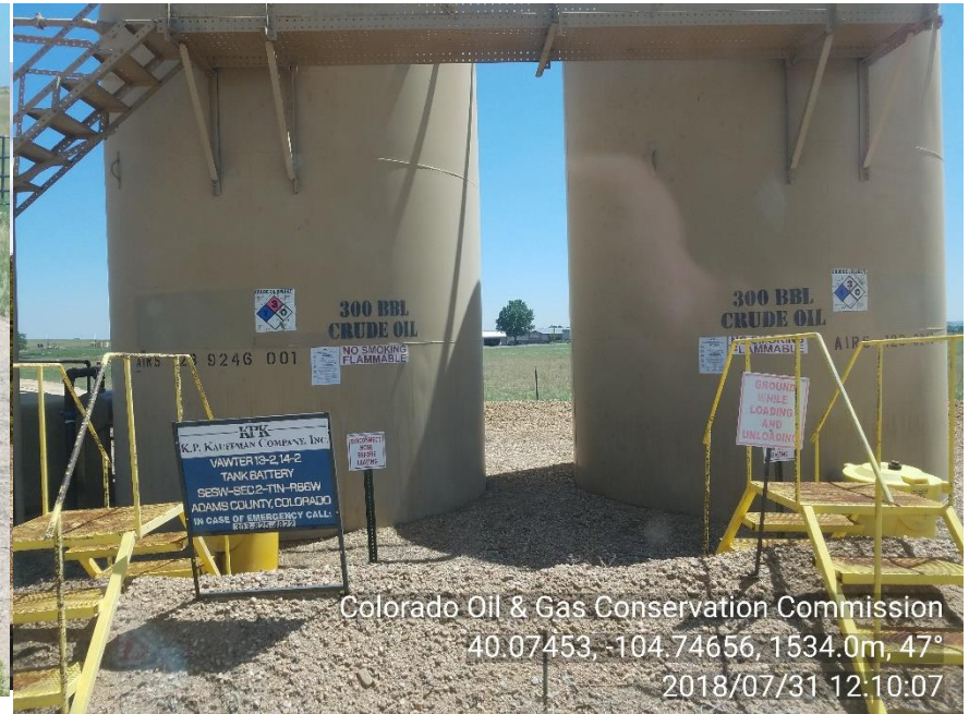
Photo 2. Tank battery
