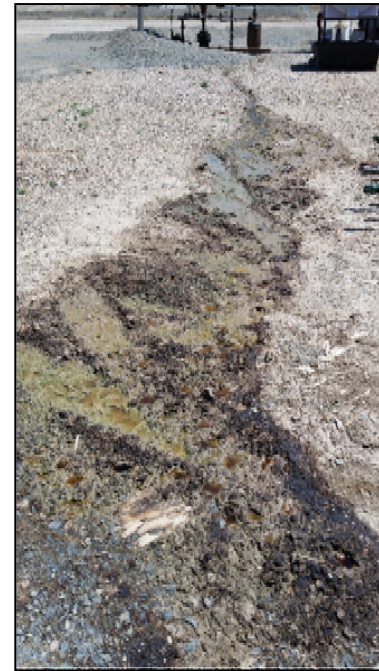
Photo 5. Drain pathway out of cellar, stained soil where fluid has evaporated.
