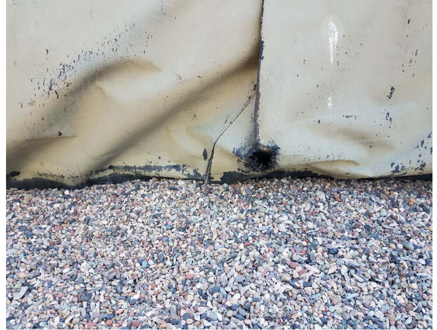
Location Photo #4, Hole in containment liner
