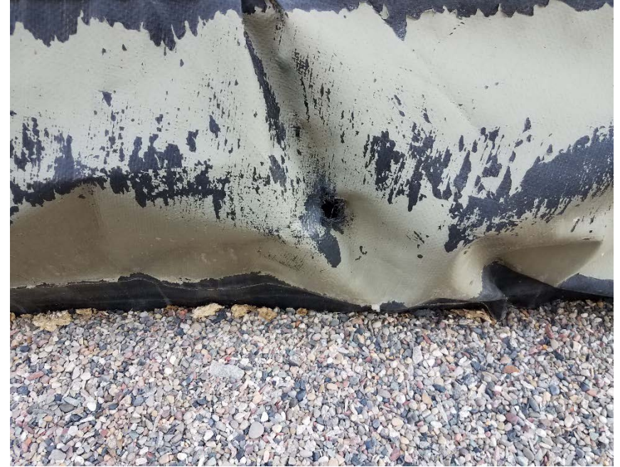
Location Photo #2, Hole in containment liner
