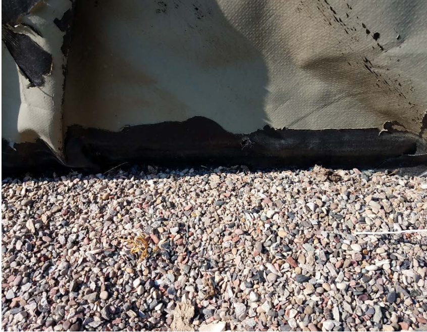
Location Photo #3, Hole in containment liner
