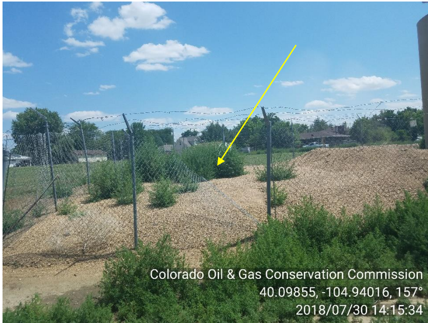
Photo 3. Fence around tank battery. Corrective action: fence down
