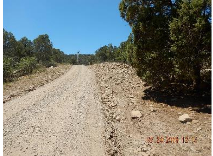
Photo 6: Access road with no stormwater velocity controls installed.
