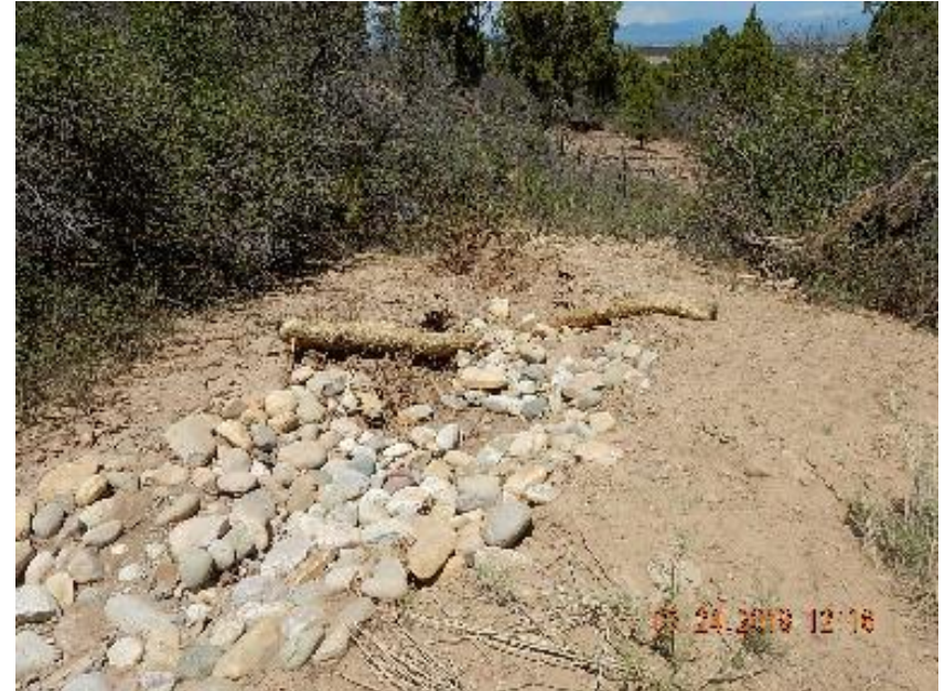
Photo 6: Blown out rip rap and waddle sediment trap on out flow of culvert.
