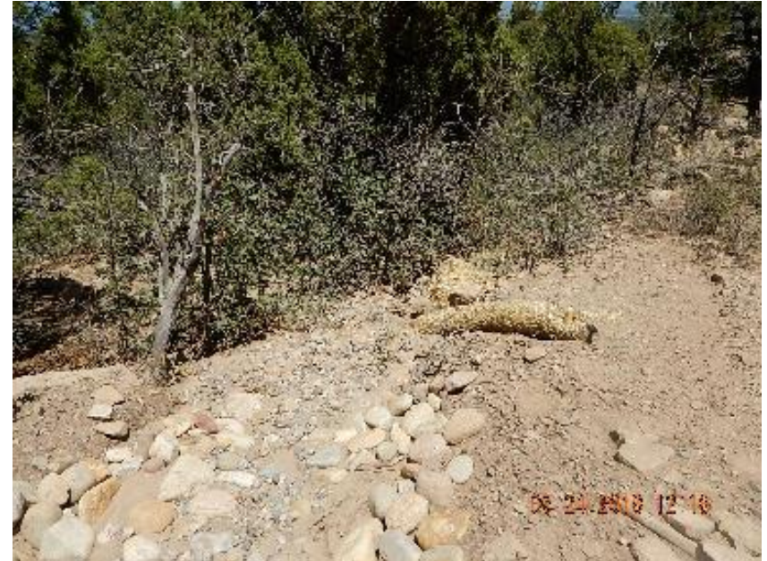
Photo 14: Blown out sediment trap, armor, and waddle.
