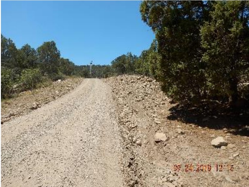
Photo 11: Access road with no stormwater velocity controls.
