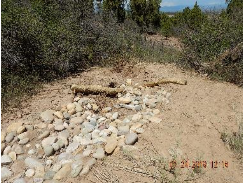
Photo 13: Blown out sediment trap.
