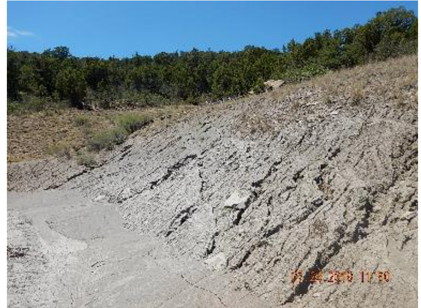
Photo 10: Rilling on cut slope with ditch at base of slope more than 75% full of sediment.
