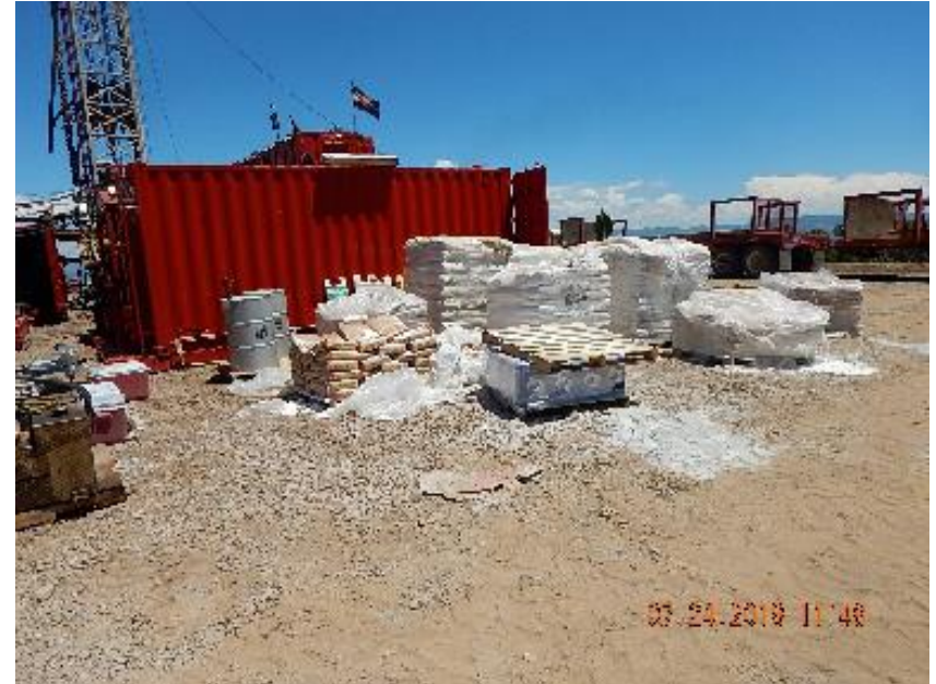
Photo 6: Spilled dry drilling materials and 55 gallon drums with no spill prevention.
