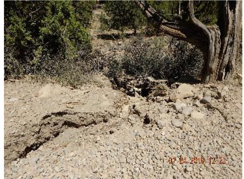
Photo 16: Stormwater flow crossing the road resulting in erosion on down slope edge of roadway.
