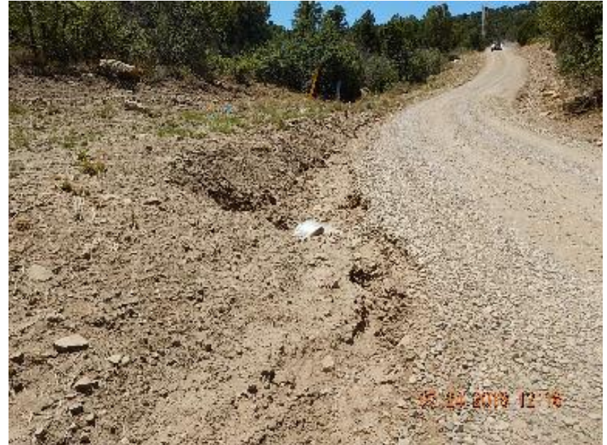
Photo 12: Stormwater flow over culvert along access road.
