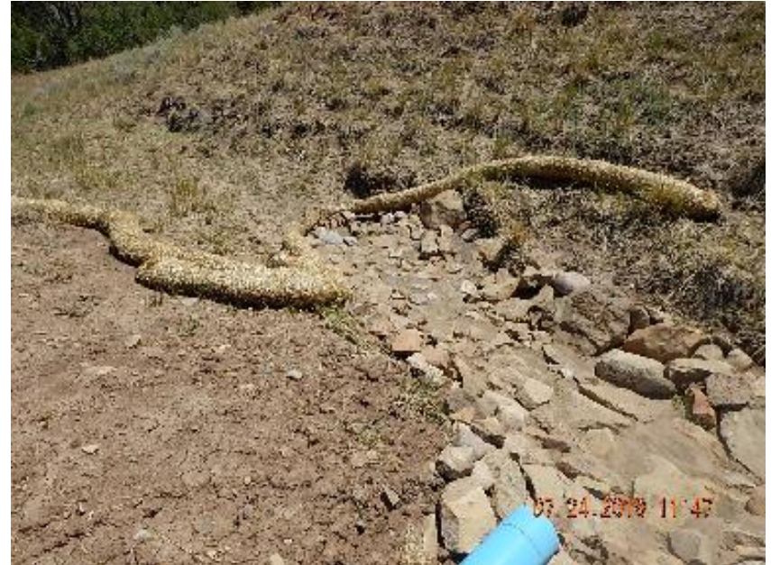
Photo 4: Waddle with stormwater flow under cutting waddle.
