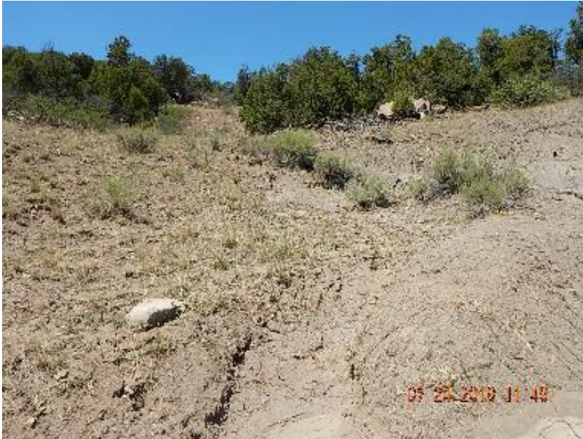
Photo 9: Breach in ditch and berm allowing stormwater and sediment to flow out of diversion ditch.
