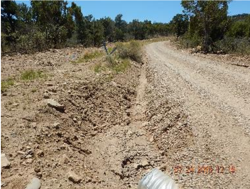
Photo 15: Ditch along access road with no storm water velocity controls.
